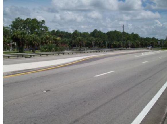
SB left-turn lane to 25 th Ave. SW (after). SB left only; no WB left.
