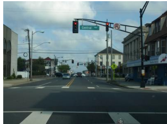
New traffic signal mast arms and signal display alignments resulting from the RSA.
