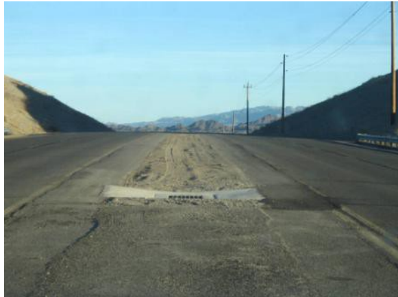
Raised traversable median drains.
