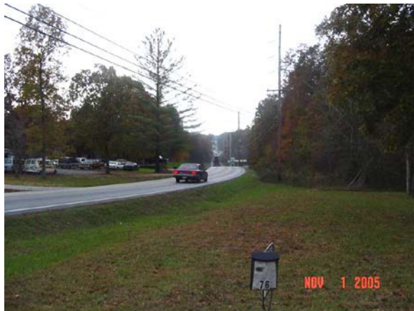
Horizontal curvature looking south at L.M. 18.50 to L.M. 18.70.
