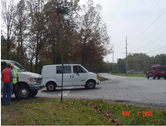
Limited sight distance looking south at L.M. 20.81.
