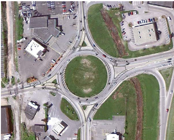
An aerial view of the City of Newport Rotary with enhanced pavement marking plan.
