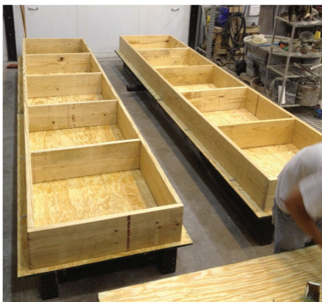
Figure 3.1 Molds for ten 3' × 3' × 10" slabs.
