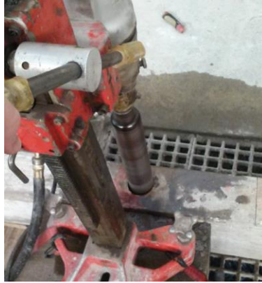
FIGURE 3.14 Coring process
