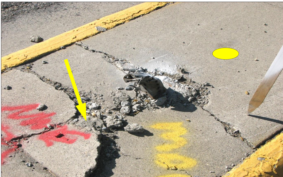
↑ ↓ Condition of the lane divider after two sign impacts. Location of the original sign placement (yellow arrow). Yellow circle will approximate location of new sign base.
