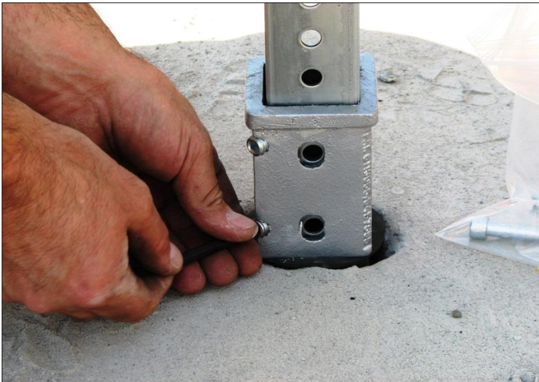
← Corner hex screws are tightened first.
