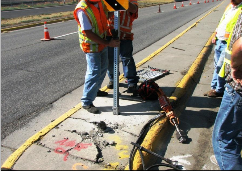
← The sign post is inserted into the Break-Out receiver.
