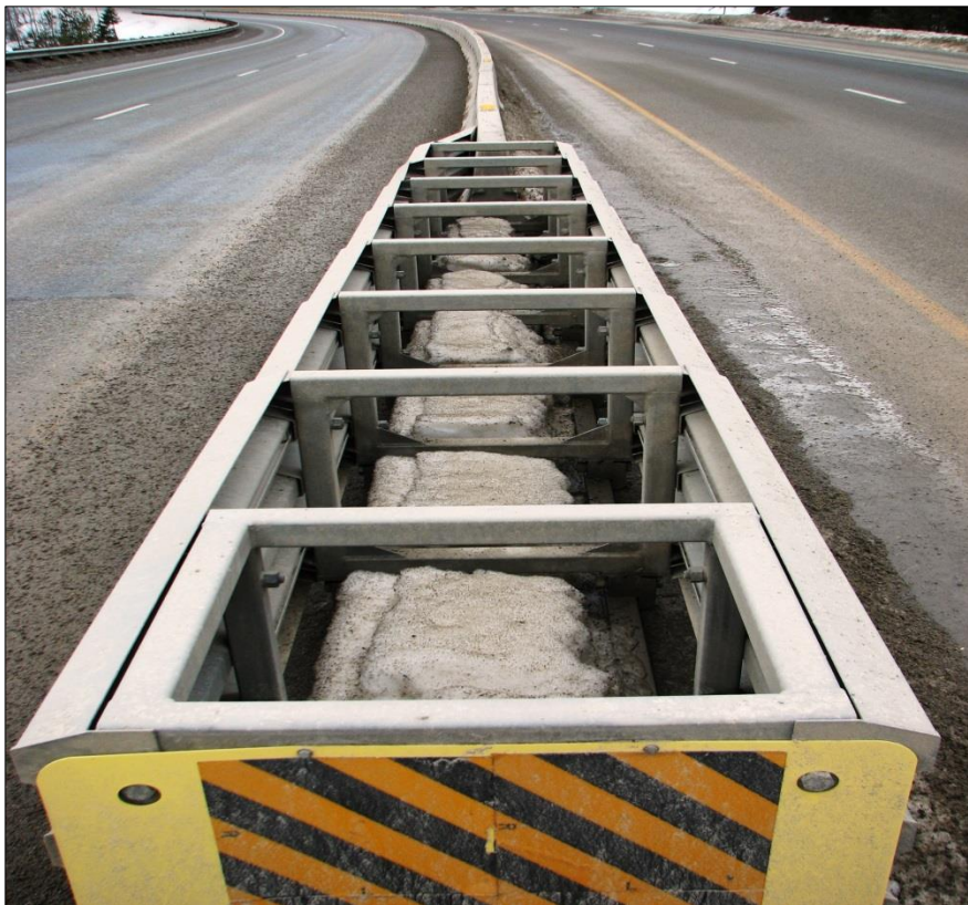
← SCI crossover installation at approximately mile point eight (8), view west.
