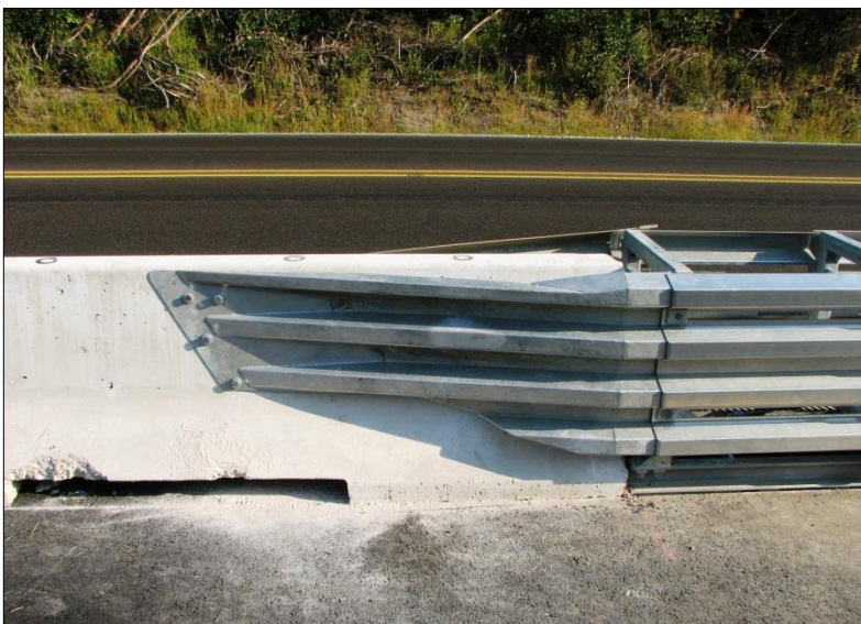
←View of completed transition panel for the F type jersey barrier.
