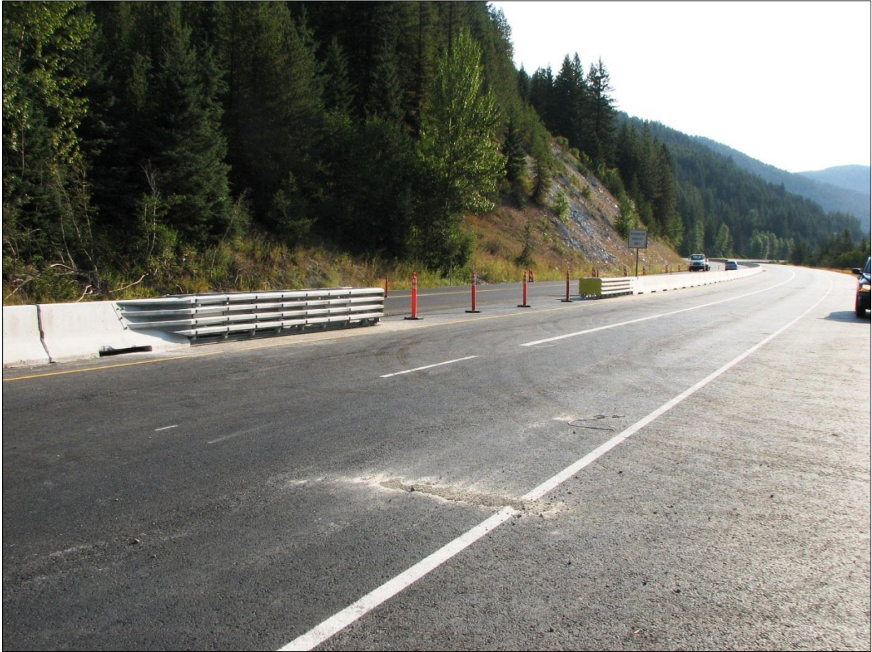
↑ Completed installation at crossover.
