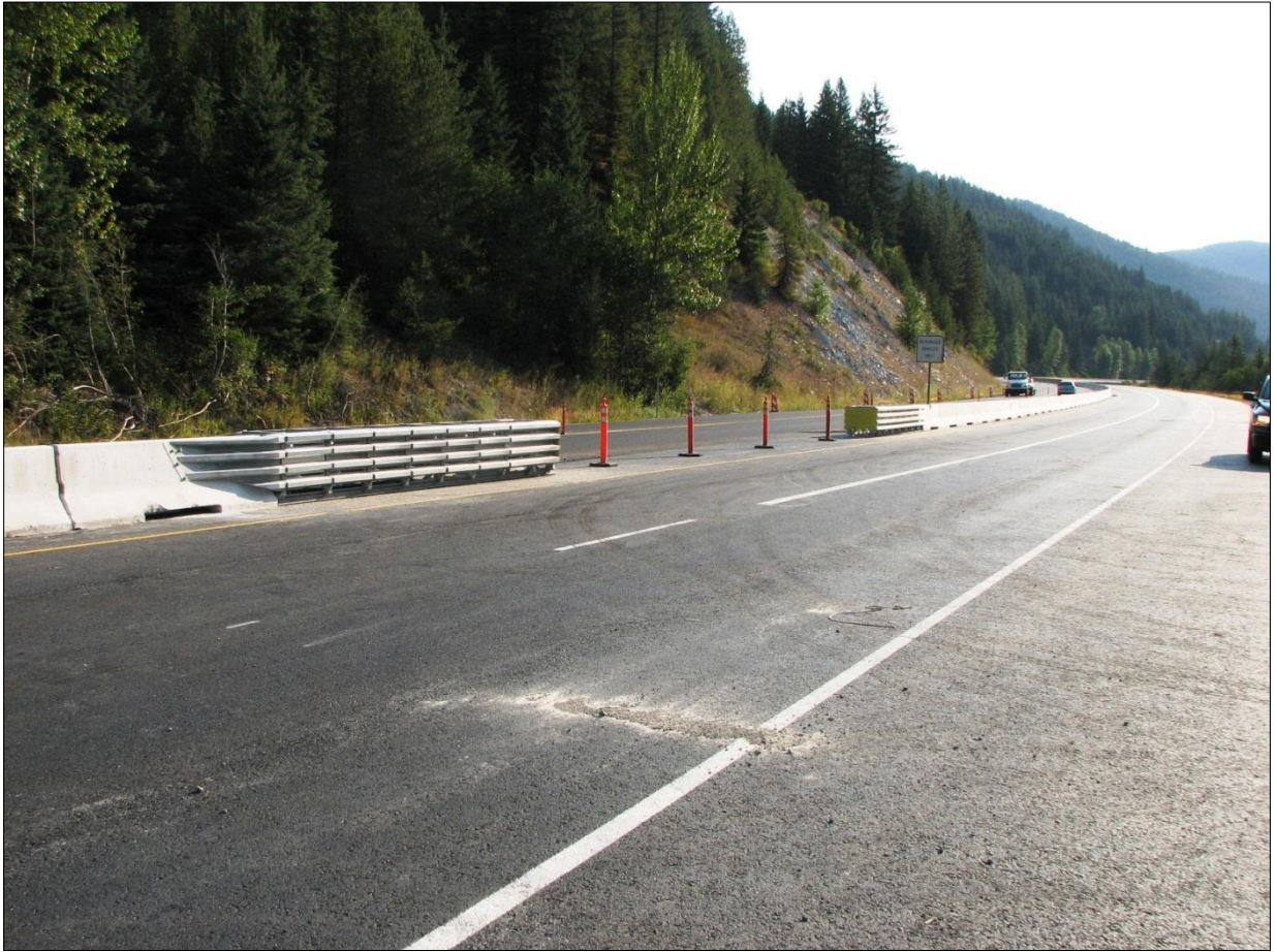
↑ Completed installation at crossover.
