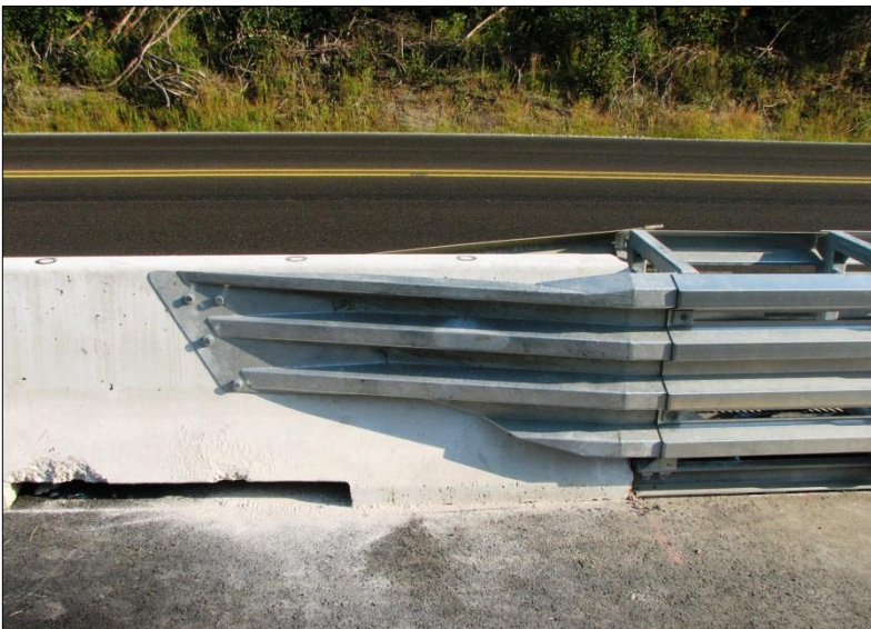
←View of completed transition panel for the F type jersey barrier.
