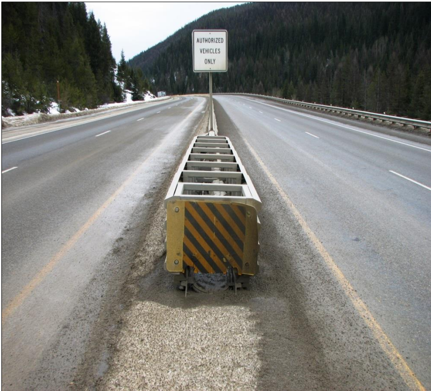
← SCI crossover installation at approximately mile point eight (8), view east.
