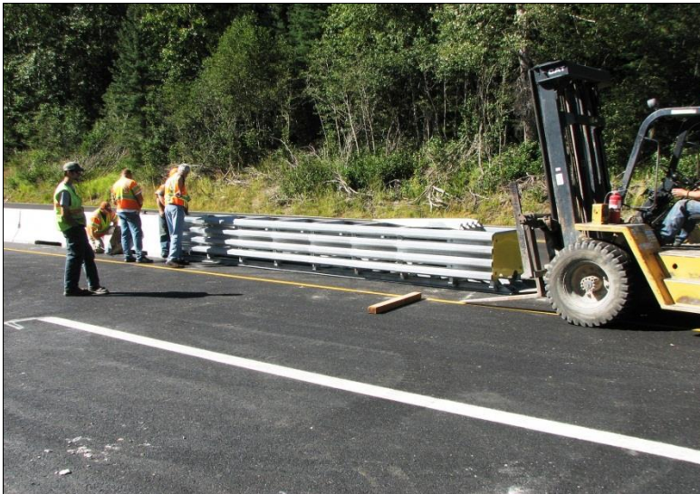
← The fork lift, at the front of the attenuator, uses its fork blade to finish the alignment.
