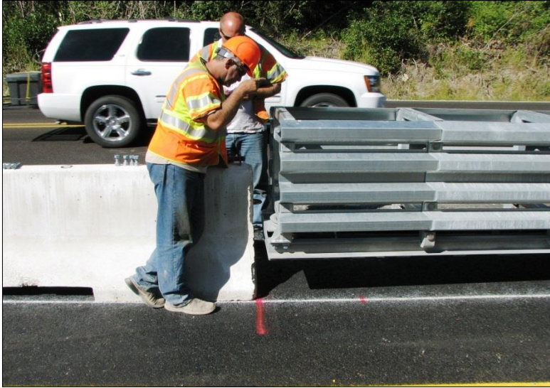
← A workman guides the fork lift operator to correct placement of the crash barrier.
