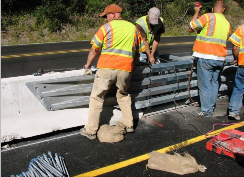
← The transition panel is being positioned for attachment to the jersey barrier and attenuator frame.
