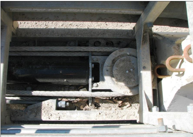
← Representative view of SCI rear mobile sheave assembly and hydraulic cylinder.
