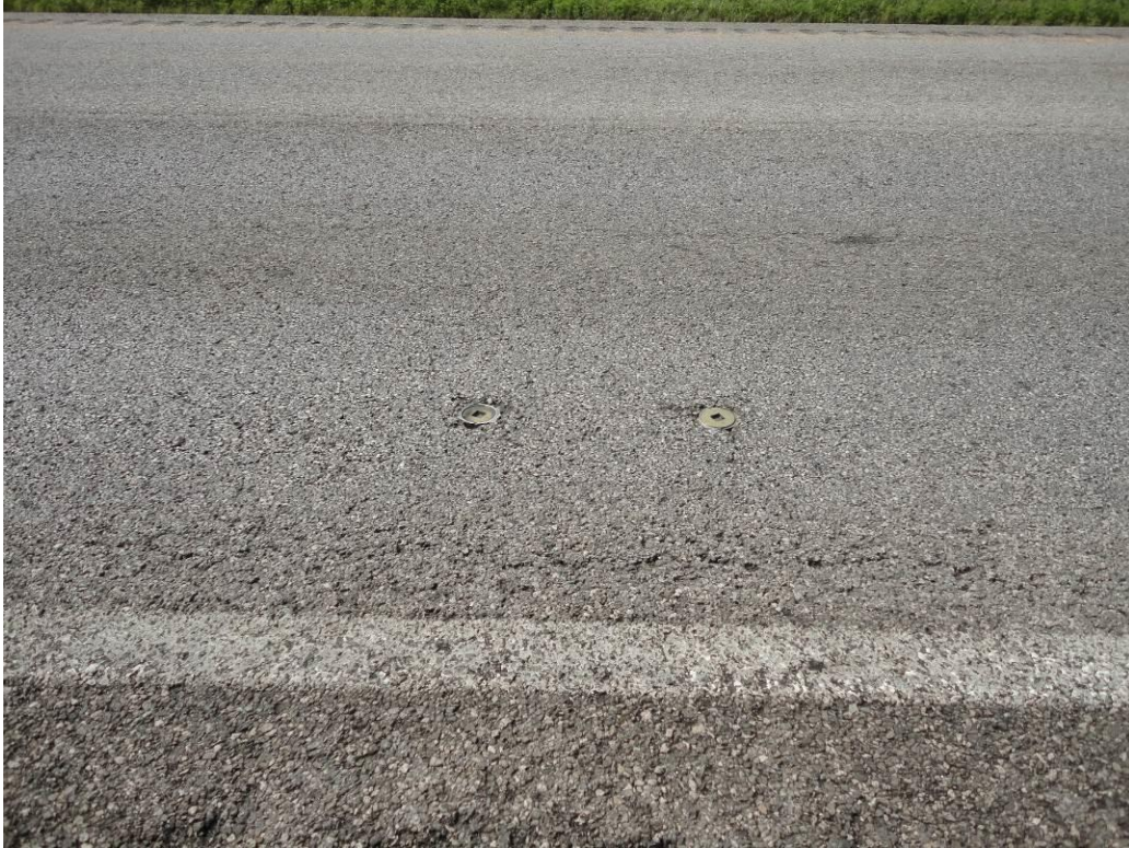
Figure 110. Test section at Sta. 664 of WAY-30.
