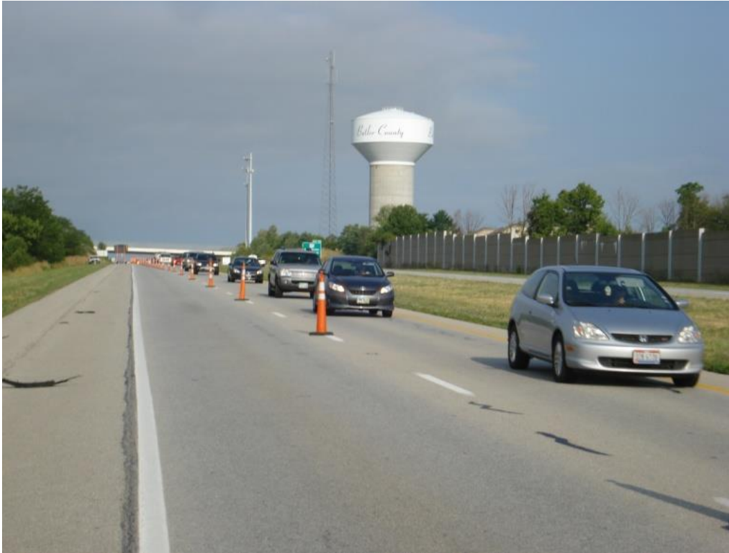
Figure 90. General view of BUT 129-22E.
