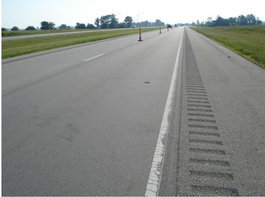
Figure 84. General view of GRE 35-21E site.
