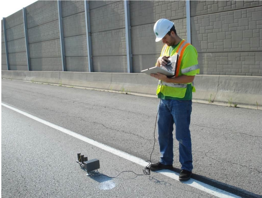
Figure 96. Field operation of the PSPA on asphalt pavement.
