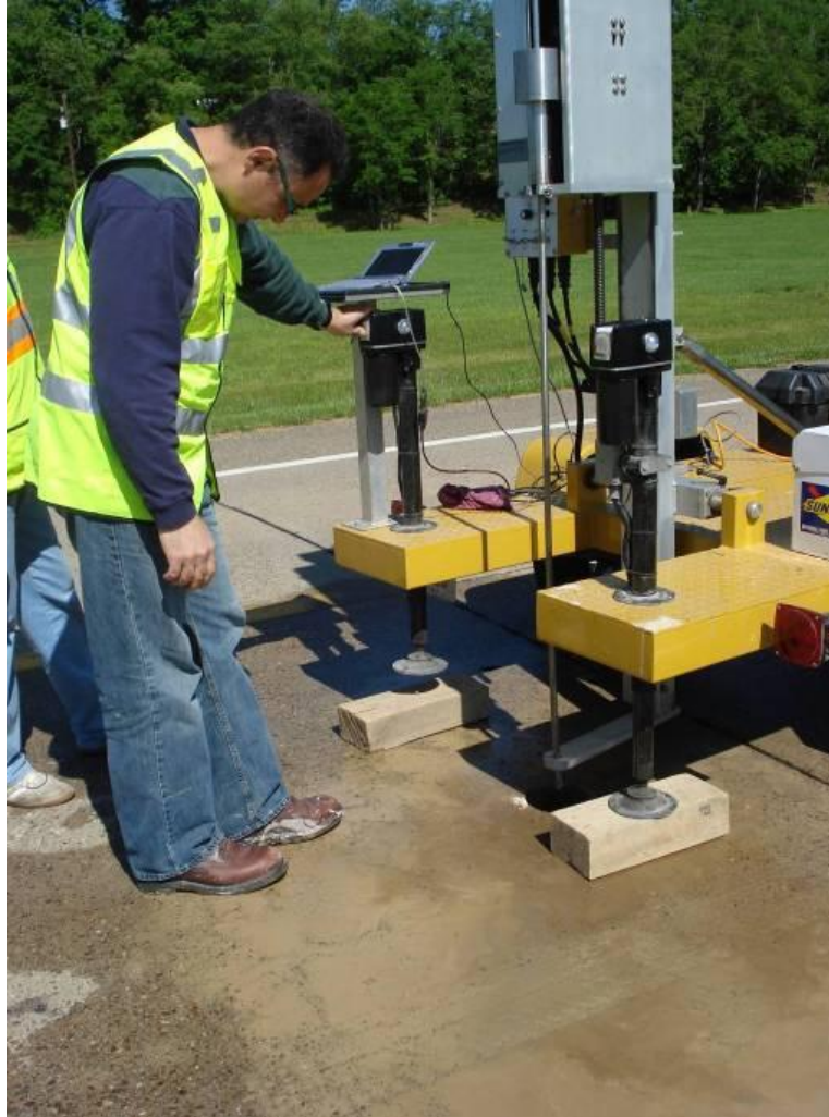
Figure 94. Automated DCP in operation.
