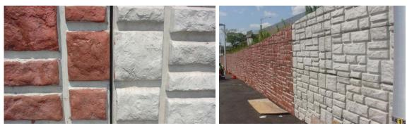
Figure 2. Contrast between Parent and Coated Surfaces
