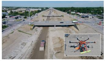
A Michigan-made unmanned hexacopter (inset) can gather aerial data quickly, like high-resolution imagery of this construction project on I-96 in Livonia.
