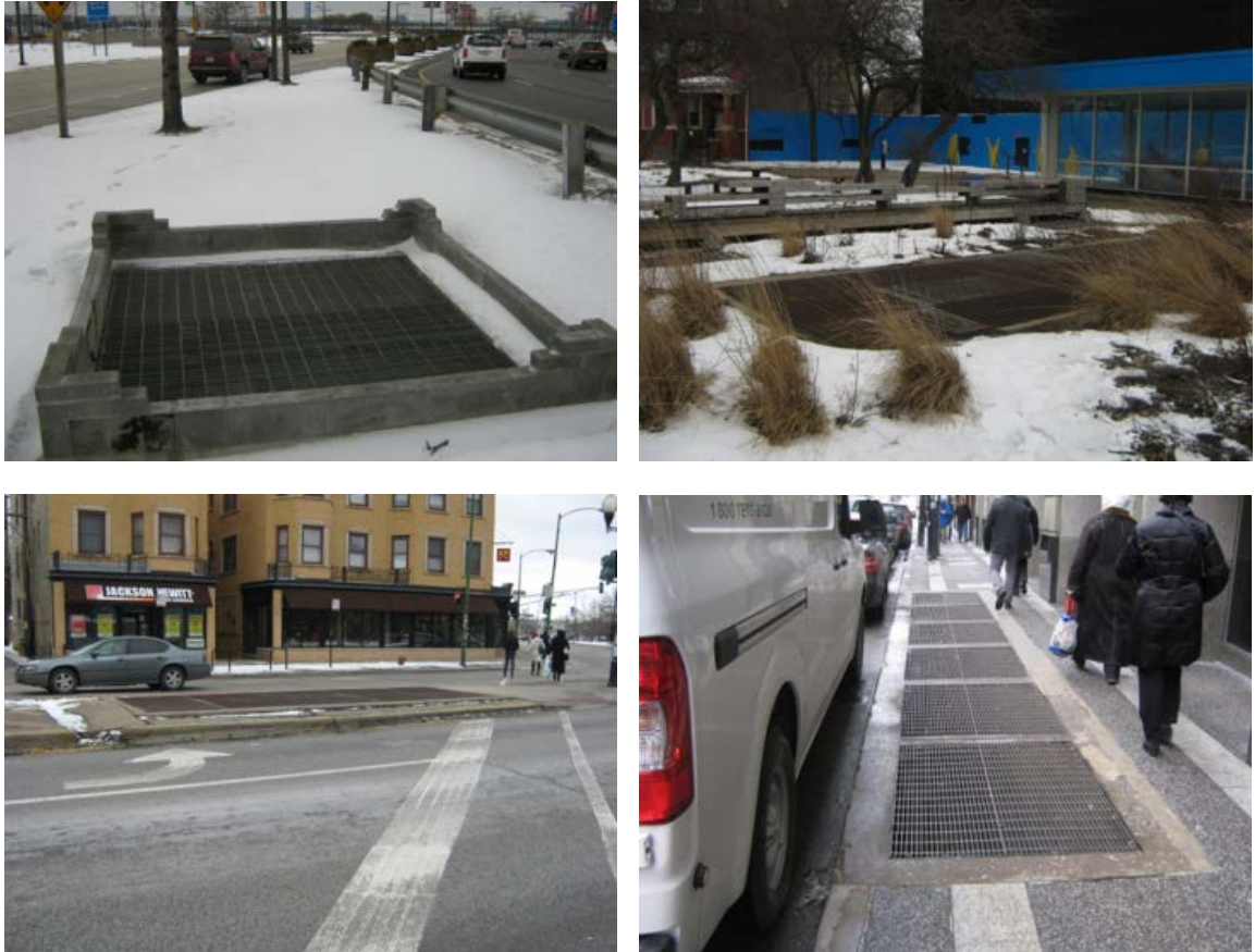
Figure 2-2 Examples of Ventilation Shafts: O'Hare Highway Median (top left), Logan Square Pocket Park (top right), Logan Square Street Median (bottom left), State Street Sidewalk (bottom right).
