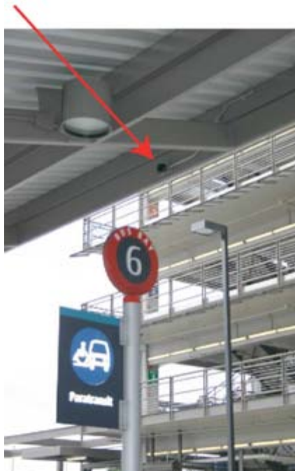
Figure 2-4 Talking Signs transmitter for Bus Bay 6 at Federal Way Transit Center
