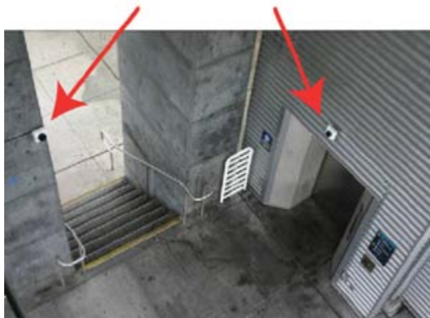
Figure 2-5 RIAS transmitters in this area of Kent Station identify and locate elevator to pedestrian bridge and stairs down to street crossing that leads to shopping center
