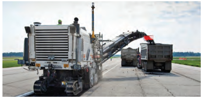
Figure 4-9. Stringless technology mounted on a milling machine.
