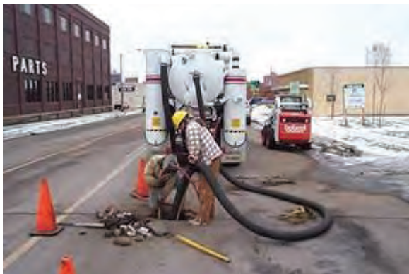
Figure 2-25. Hydro excavation operation to locate underground utilities.
