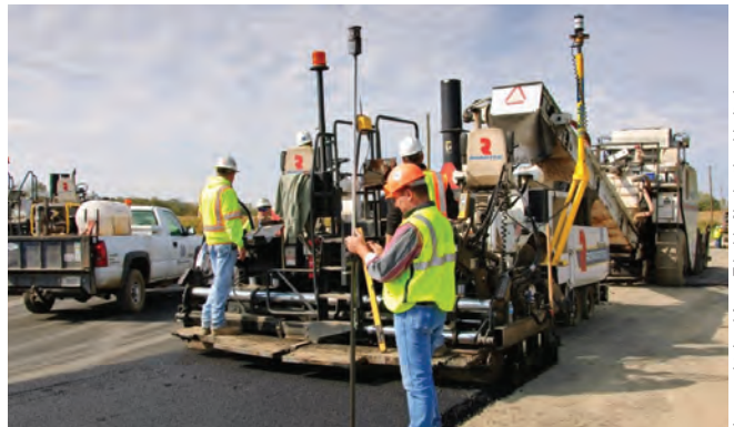
Figure 4-8. Stringless paving can be used for asphalt applications in addition to concrete.
