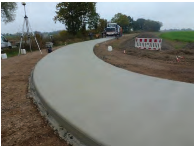
Figure 4-13. A horizontal curve that was paved using stringless technology.
