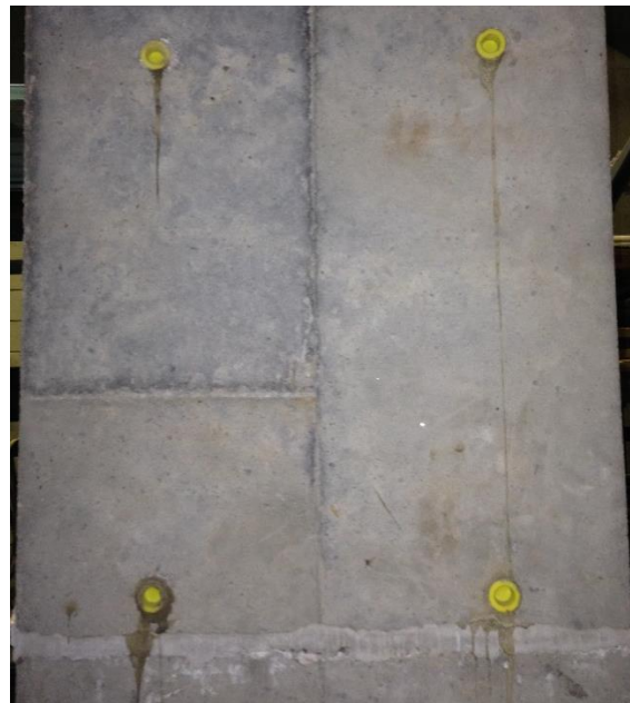
Figure 14. Port plugs installed after grouting
