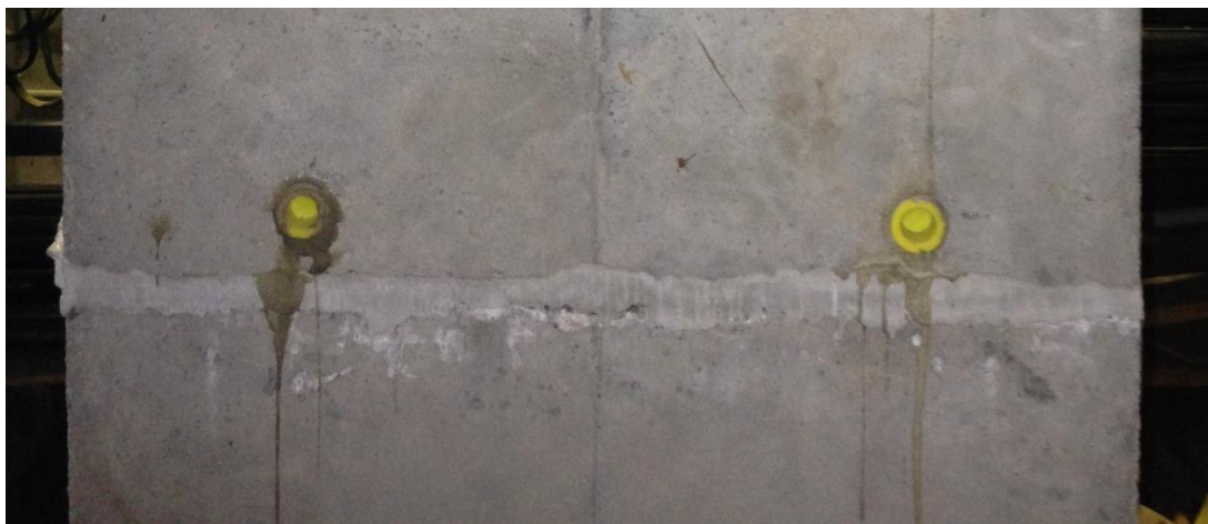
Figure 10. Specimen grout bed using UHPC
