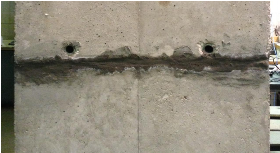
Figure 9. Specimen grout bed using W. R. Meadows 588-10k
