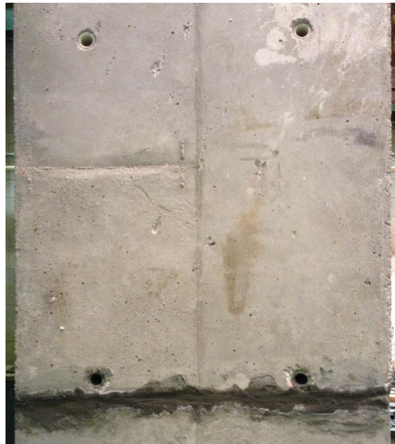
Figure 13. Port plugs before grouting
