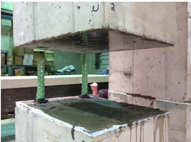
Sleeve-lock seal plugs were used on protruding reinforcing steel to keep bedding grout from entering couplers, grout was placed on top of the bottom specimen, and top specimen was carefully lowered on top
