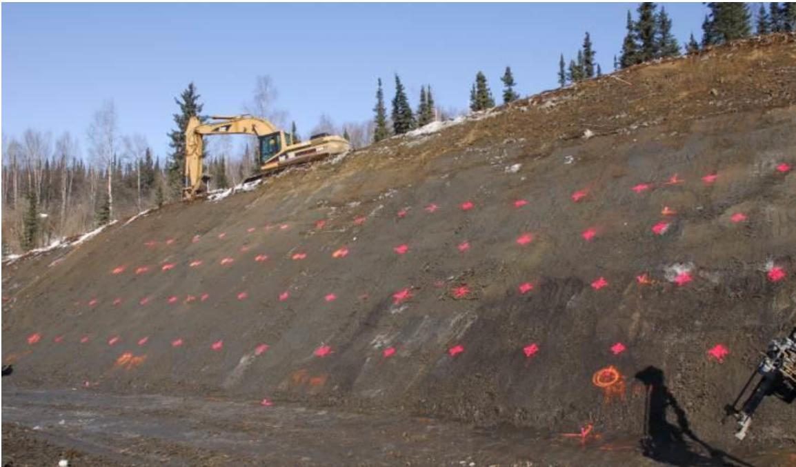
Figure 4.2 Layout on the cut slope
