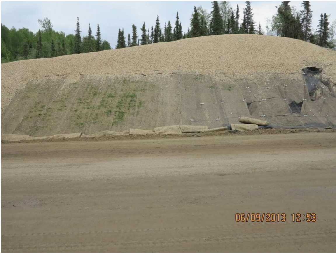
Figure 6.4 Surface protection matting in area showing no grass growth is not in direct contact with ground surface
