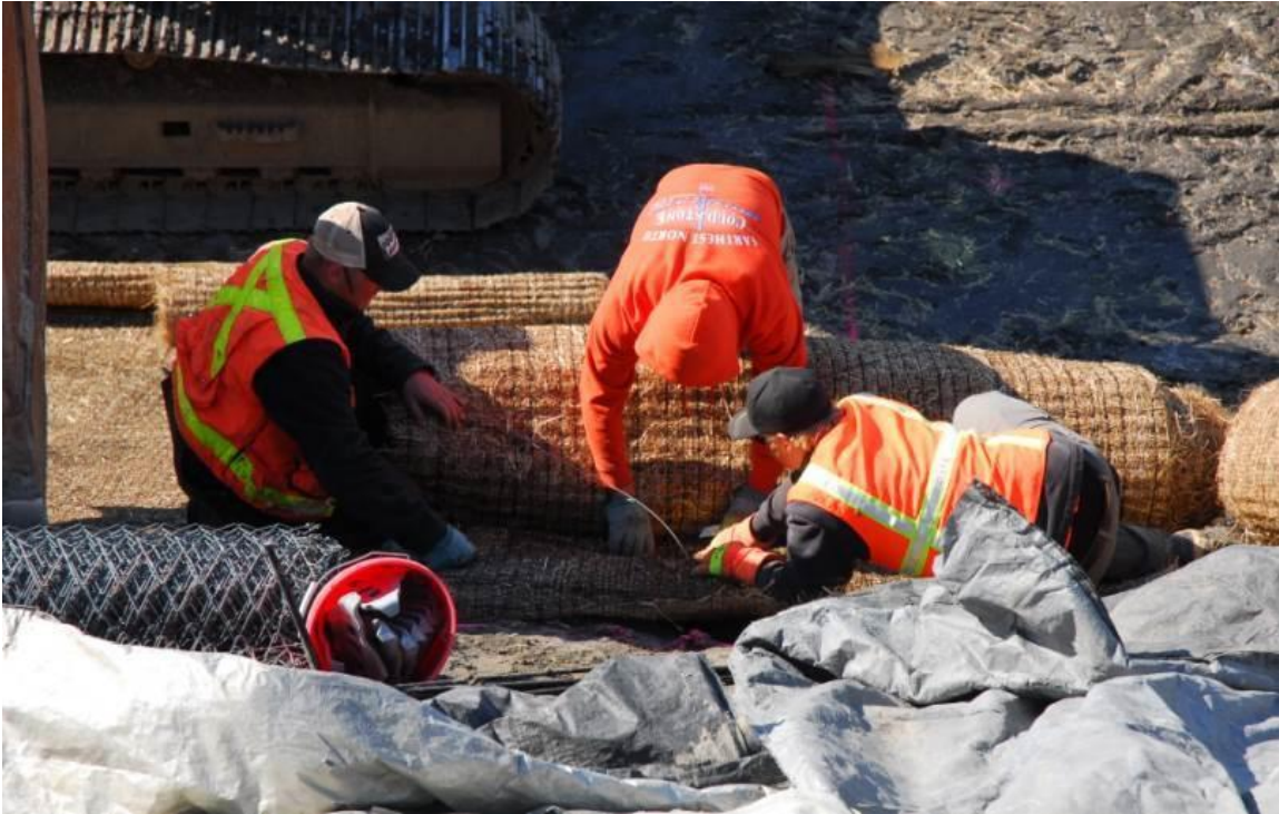
Figure 4.15 Placement of the coconut erosion control matting
