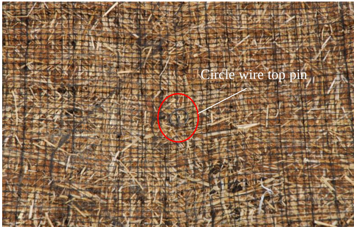
Figure 4.18 Enlargement of a circle wire top pin
