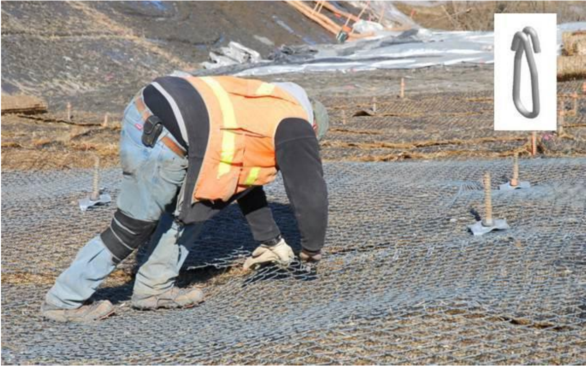
Figure 4.21 Connecting adjacent Tecco-mesh strips
