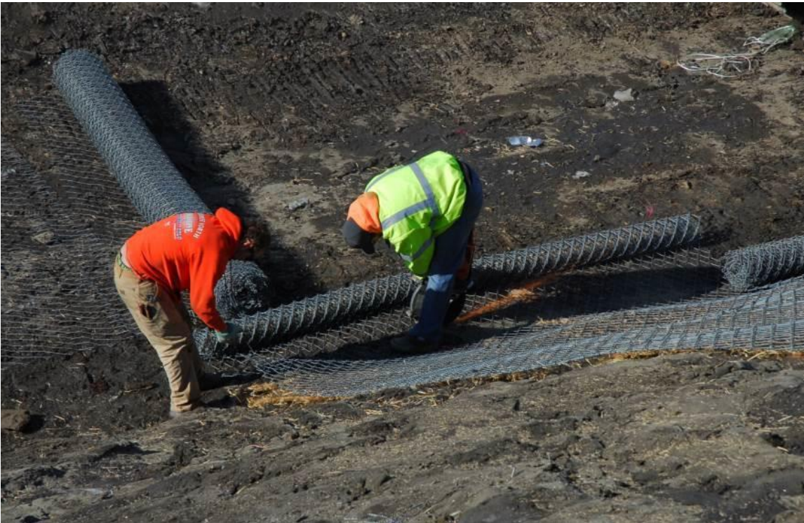
Figure 4.20 Cutting away excess Tecco-mesh
