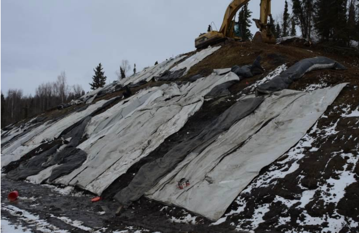
Figure 4.10 Cut slope protected from erosion during drilling
