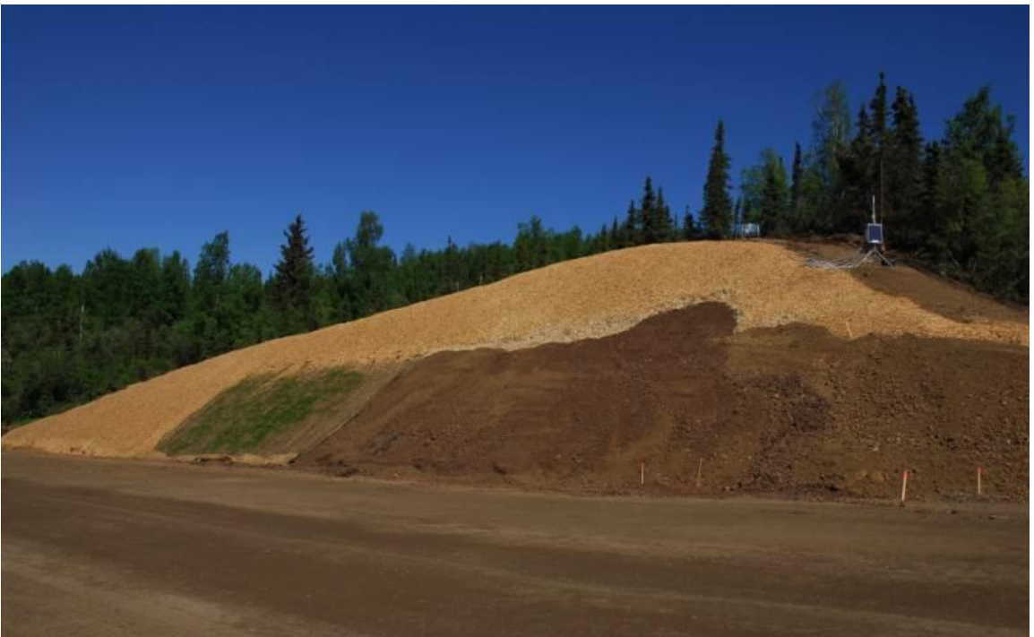
Figure 6.8 Cut slope after construction on Section C
