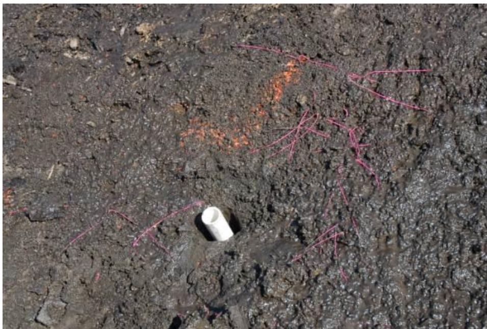
Figure 4.6 Instrumentation hole with sensor housing installed
