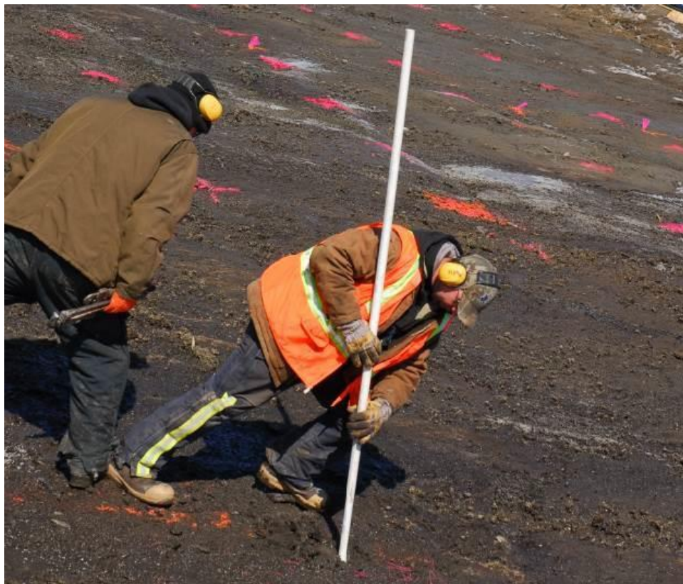
Figure 4.5 Installation for sensor housing
