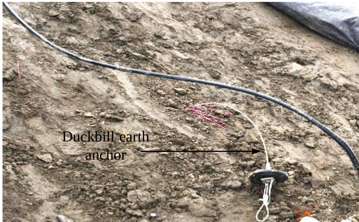
Figure 4.11 Cable end of installed duckbill earth anchor
