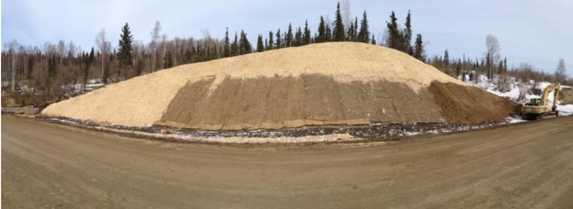
Figure 4.26 Appearance of Experimental Feature soon after completion
