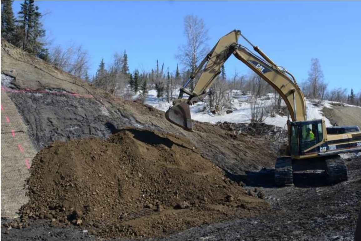
Figure 4.24 Construction of Section D
