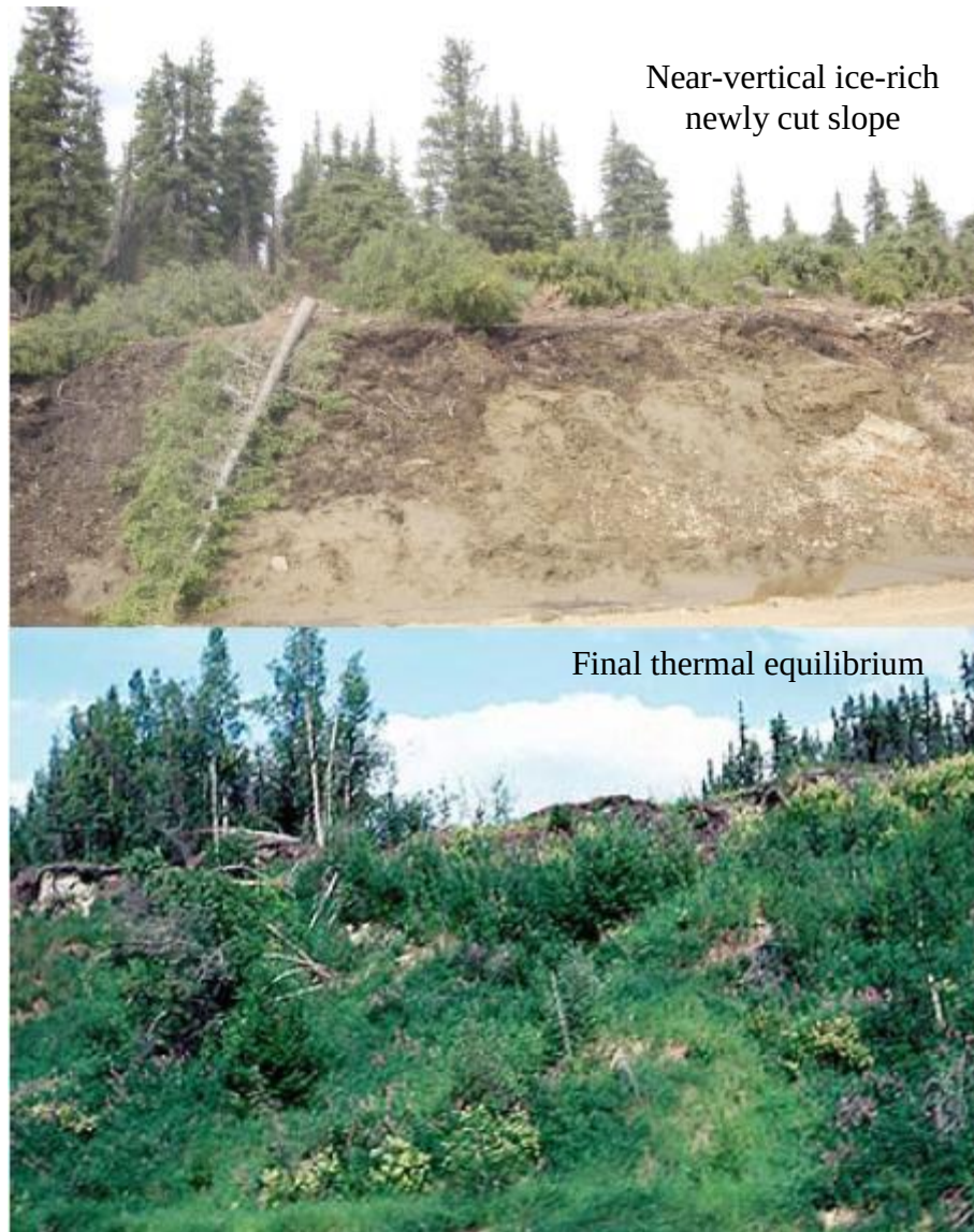
Figure 2.1 Ice-rich cut slope (Mageau and Rooney, 1984)
