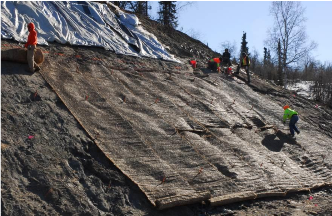
Figure 4.16 Placement of coconut erosion control matting
