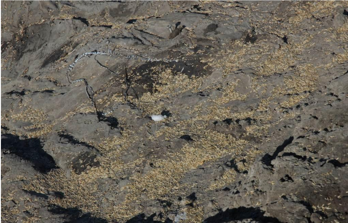
Figure 4.14 Seeded cut slope
