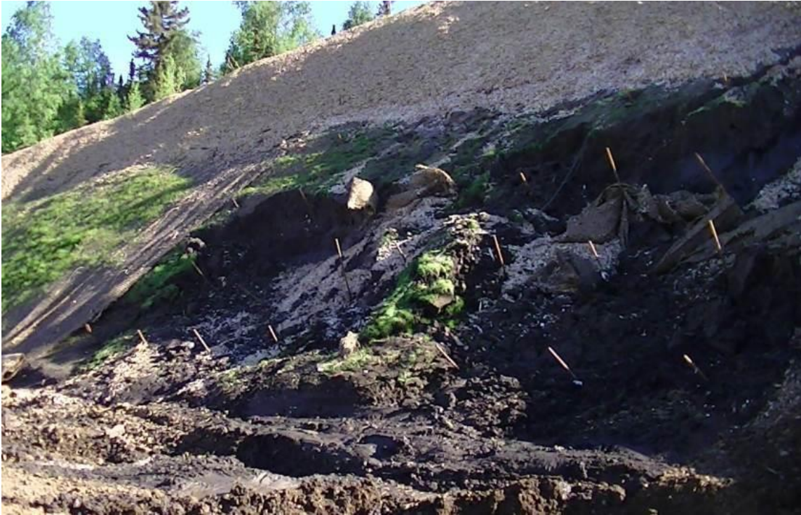
Figure 6.5 Section C without Tecco-mesh and coconut blanket
