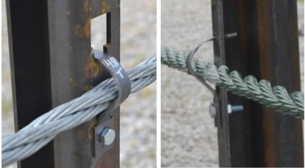
Figure 1. Bolted, Tabbed Bracket on MWP
