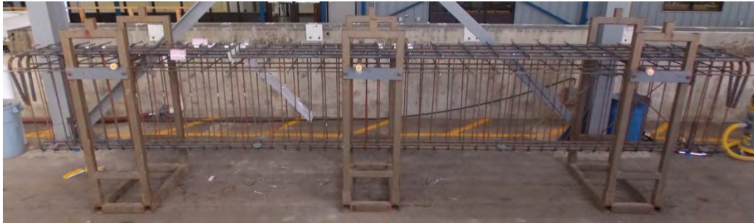
Figure 3.21: Finished rebar cage.
