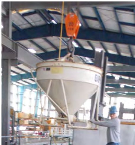
Figure 3.25: a) Clamshell bucket carrying concrete and b) consolidating concrete.
