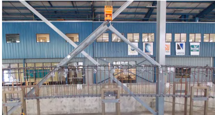
Figure 3.24: Typical cage lifting process.
