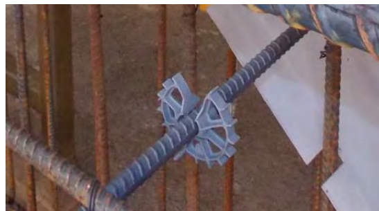
Figure 3.22: Chair used to ensure cover concrete.
