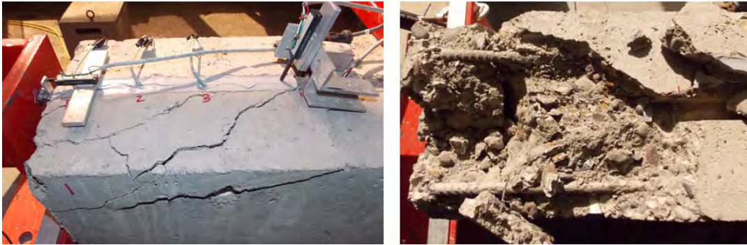
Figure 4.48: Bond stress test specimens with 12 in. bond length at failure (left) and detail of remaining concrete (right).
