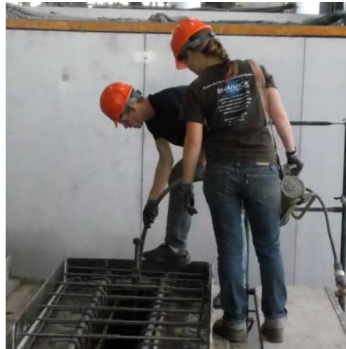
Figure 3.25: a) Clamshell bucket carrying concrete and b) consolidating concrete.
