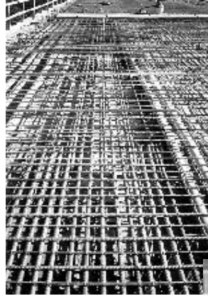
Stainless steel rebar on the Haynes Inlet Slough Bridge deck.
