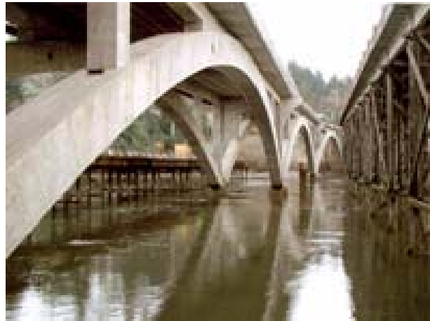
Haynes Inlet Slough bridge, Oregon
