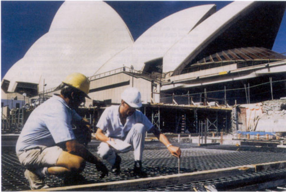
Sydney Opera House, ANCON CCL, UK
