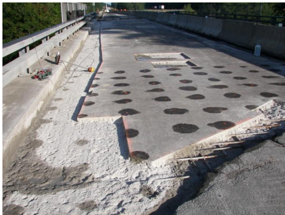
South curb concrete removed
