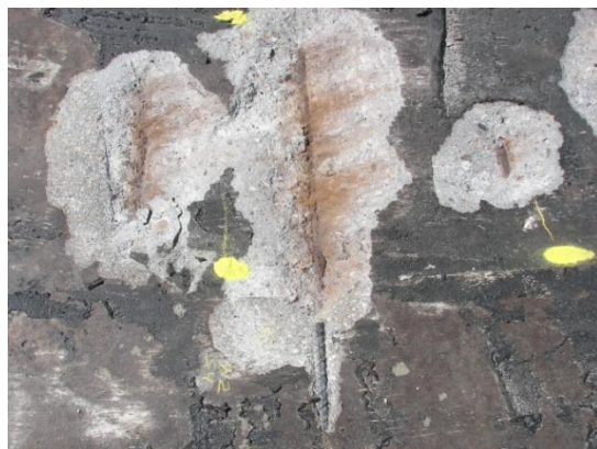
Figure 2. Anodic and cathodic rebar
