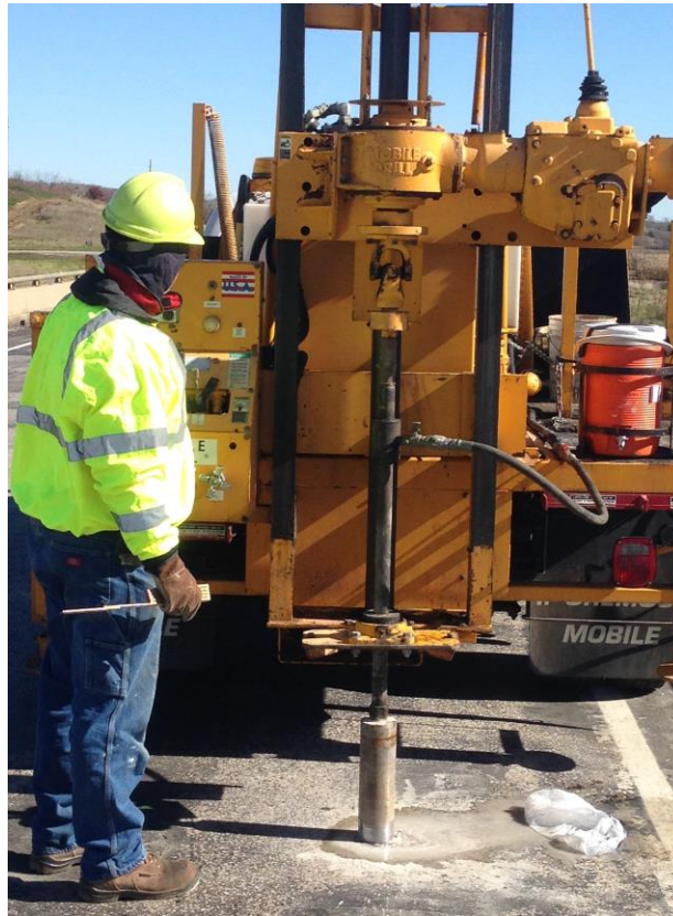
Figure 51. Drilling equipment attempting to core the concrete bridge deck
