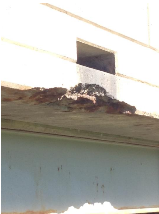
Figure 38. Close up of thickness of concrete bridge deck
