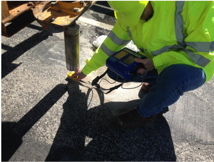
Figure 50. Steel locator being used by MoDOT technician
