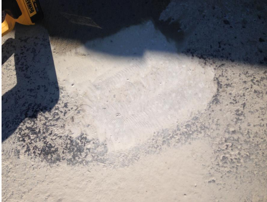
Figure 45. Ground spot where asphalt emulsion was beforehand
