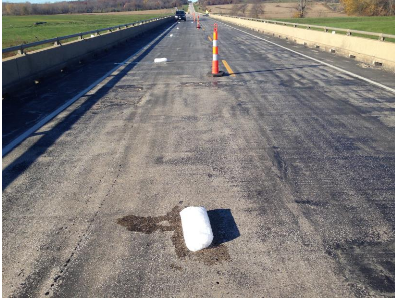
Figure 44. View of ice bags facing west on the bridge
