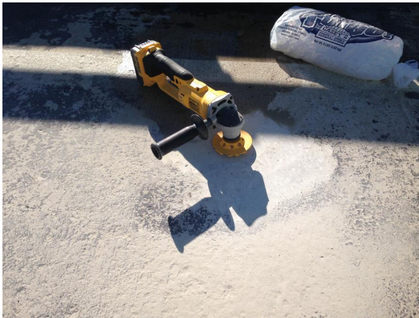
Figure 46. Angle grinder shown in a previously ground spot of pavement
