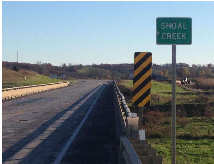
Figure 34. Shoulder view of bridge looking east
