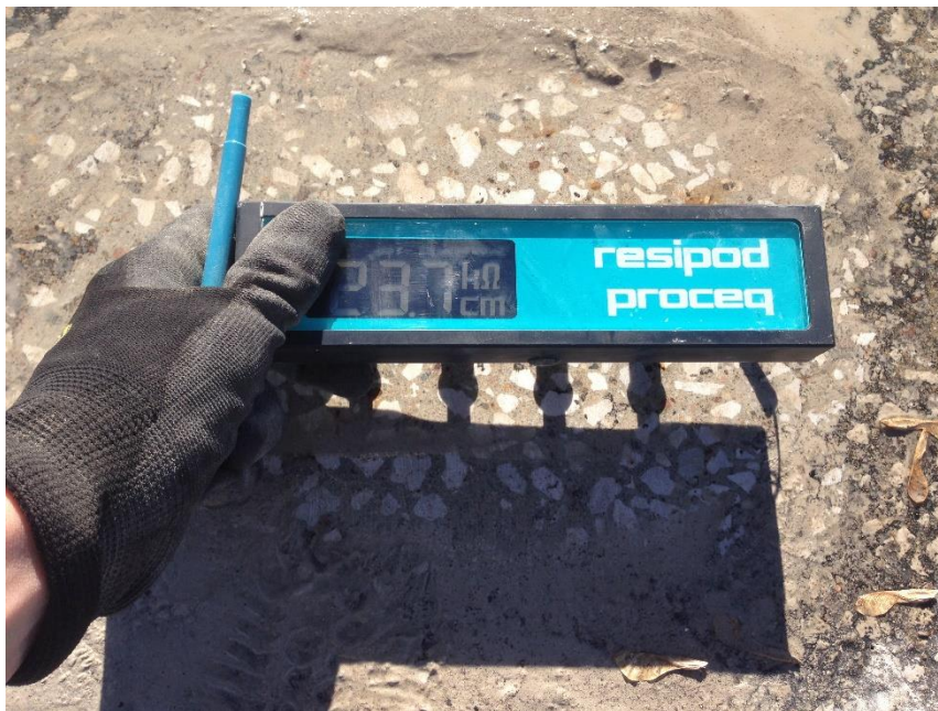
Figure 49. Surface resistivity testing on the bridge deck
