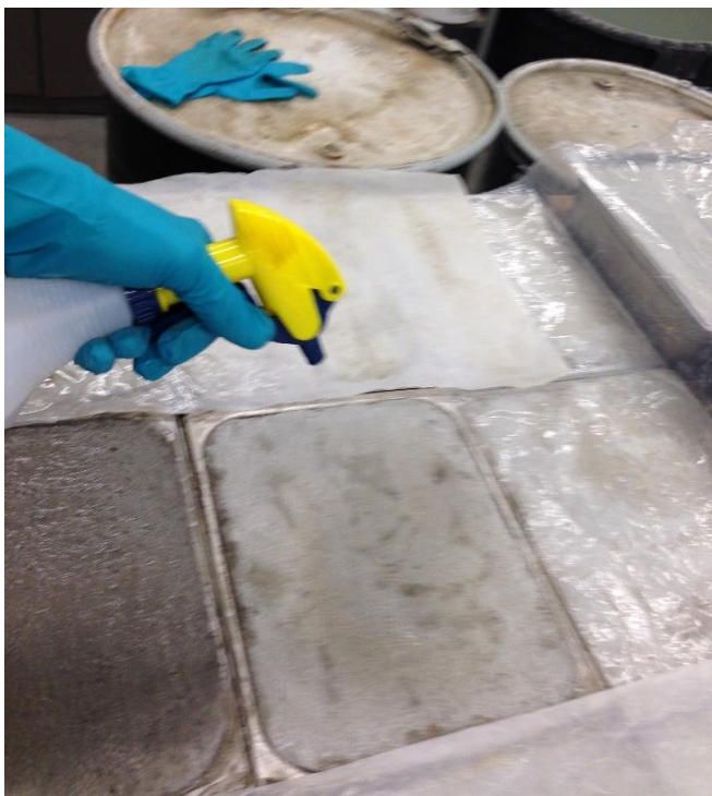
Figure 55. Sealer being sprayed and applied to concrete
