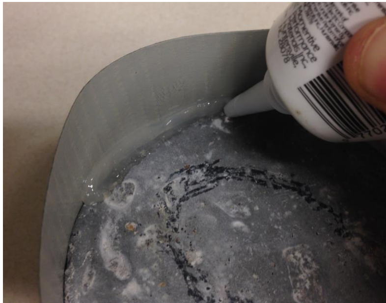
Figure 13. Caulking the joint between concrete and tape
