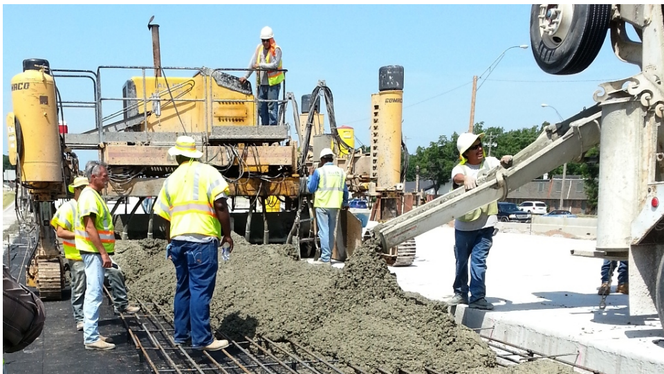
Figure 17 - Casting the concrete pavement
