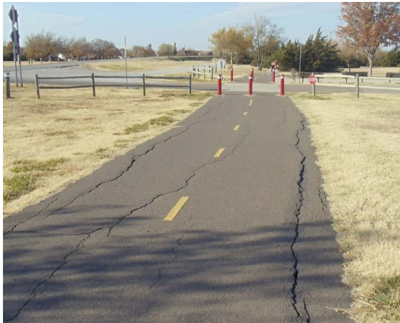
Figure 3.1. Longitudinal Drying Shrinkage Problem at Norman Site (Photo taken on November 21, 2012).
