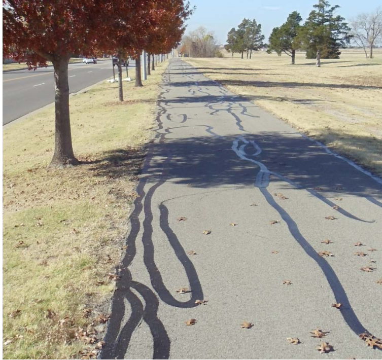
Figure 3.1. Longitudinal Drying Shrinkage Problem at Norman Site (Photo taken on November 21, 2012).
