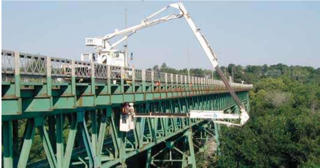
Figure 67: Inspectors use an under-bridge inspection vehicle during an In-Depth Inspection (STRUCTUREmag.org).
