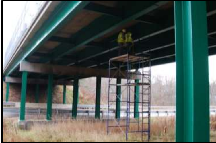
Figure C-5: Scaffolding Assembled at Bagdad Rd Installation Site
