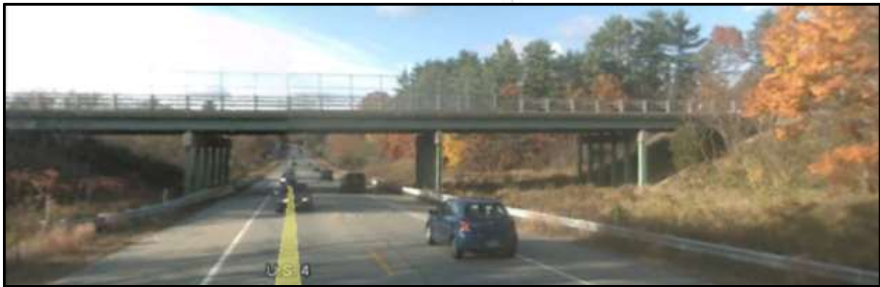
Figure 15 Bagdad Road Over US Route 4
