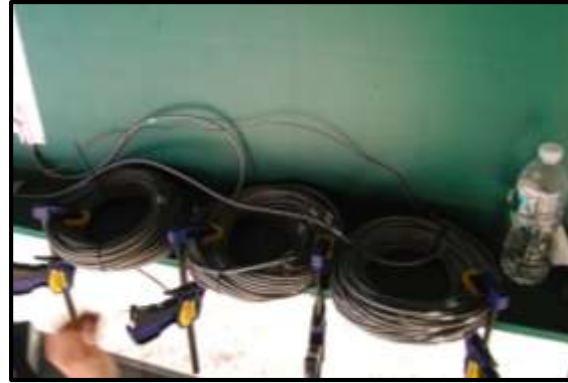
Figure C-18: Photo of Gauge Installation – Wires Clamped to Bottom Flange
