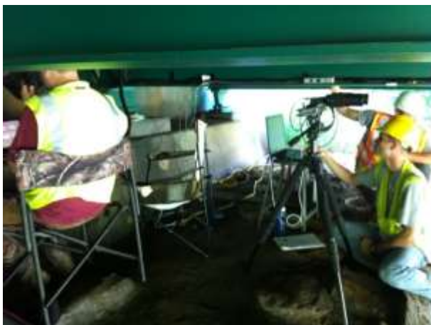
Figure 41: Camera system setup beneath Bagdad Road Bridge for load test.
