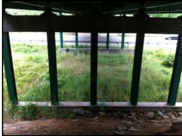
Figure 23: Photo of the Underside of Span 3 Viewed from Under Span 4
