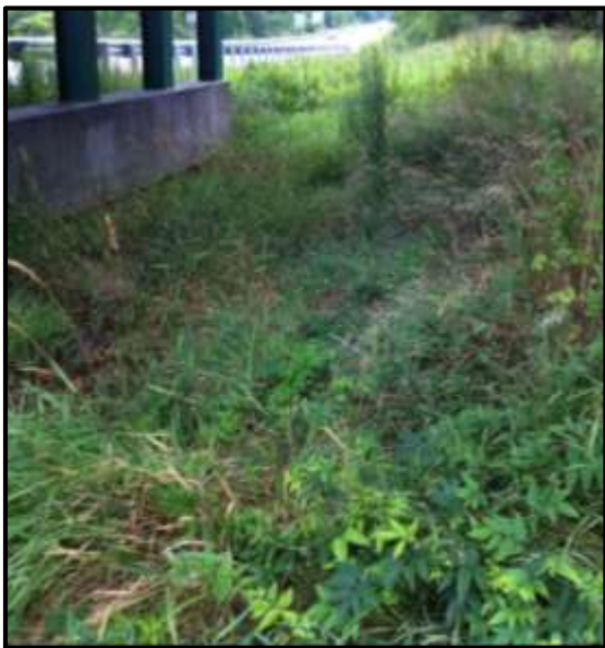
Figure C-1: Photo of Ditch Between Roadway and Underside of Span 3 at BRB
