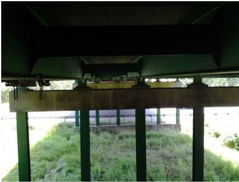
Figure 42: Targets attached to girders. Note: targets identified by circles; not all targets are shown.
