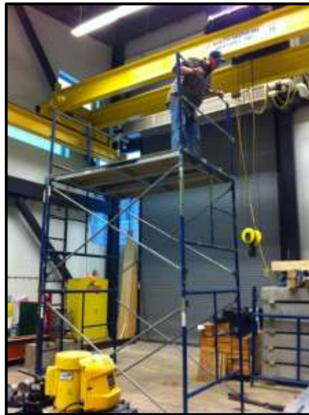
Figure C-3: Photo of Scaffolding Assembled during Practice Run
