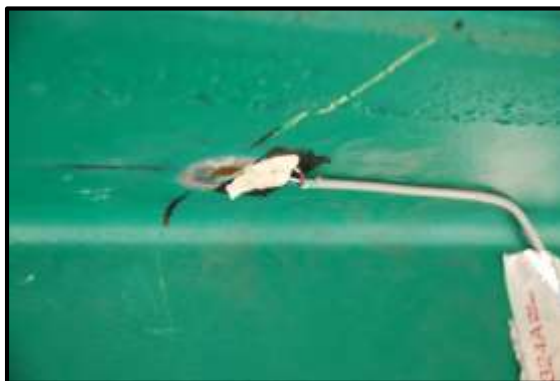
Figure C-15: Photo of Gauge Installation – Putty Placed Over Leads
