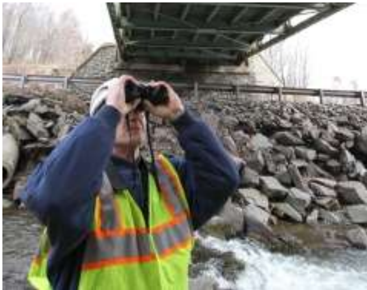
Figure 66: PennDOT inspector assesses an abutment using binoculars during a Routine Inspection (Scranton Times Tribune).
