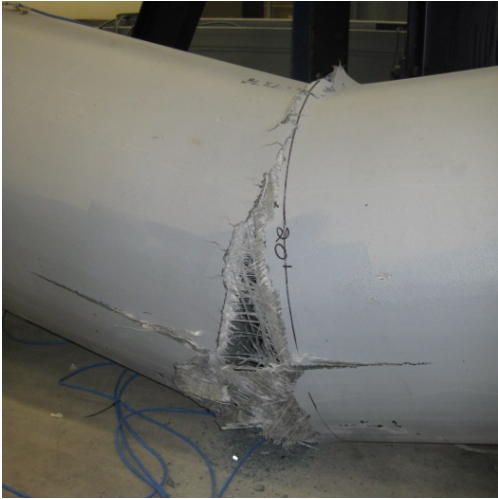
Figure 23: Tension Failure of Pile H-4FB
