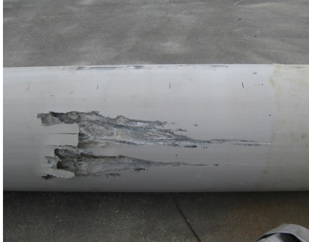
Figure 31: Hole in Pile D Due to Extraction
