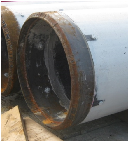
Figure 2: Driving Shoe for Hollow Piles
