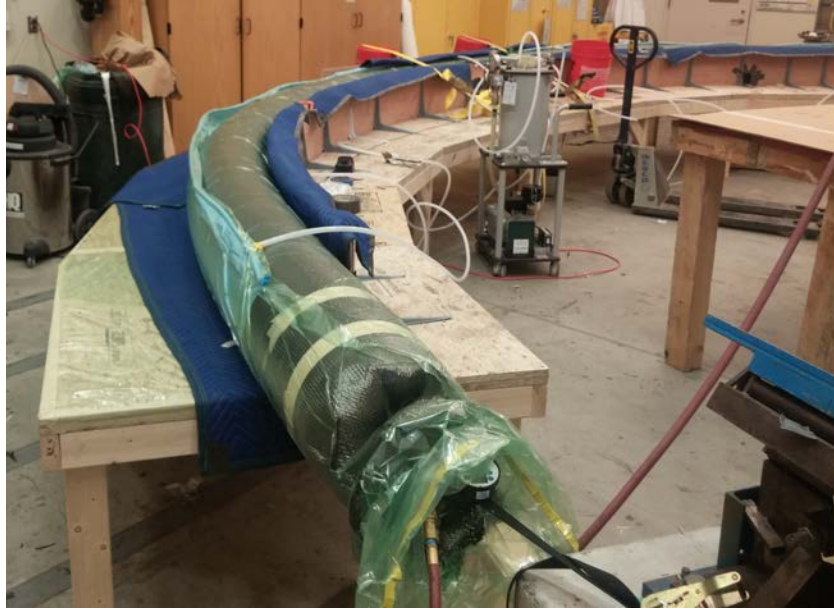
Figure 6 - Arch on formwork during infusion process
