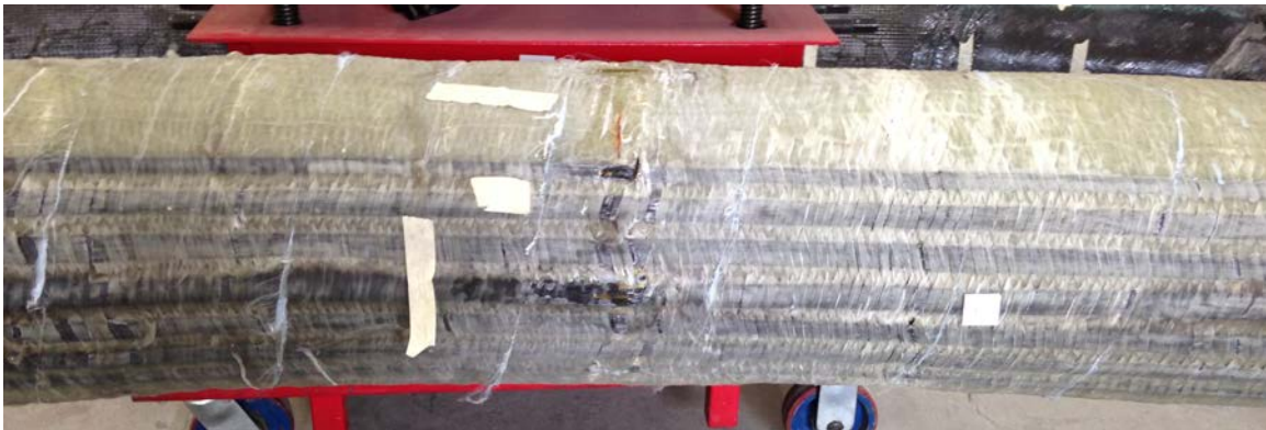
Figure 24 - Underside of midspan of arch after failure (discoloration seen on left)
