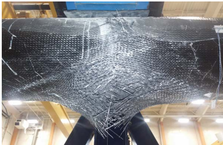
Figure 9 - Tensile rupture of FRP at crown of arch
