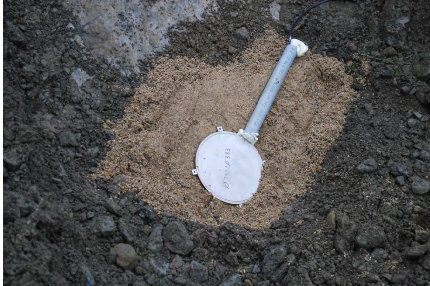
Figure 7: TPC in place prior to backfilling
