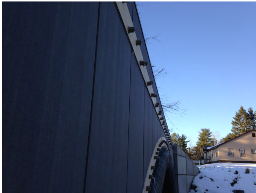
Figure 39 - Headwall of Jenkins Bridge (2014)
