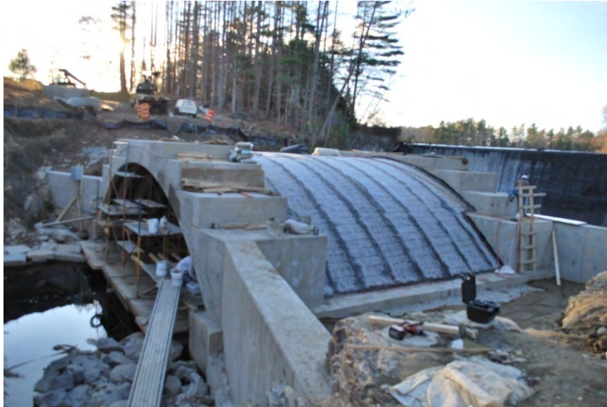
Figure 5: Perkins Bridge prior to backfilling of the superstructure
