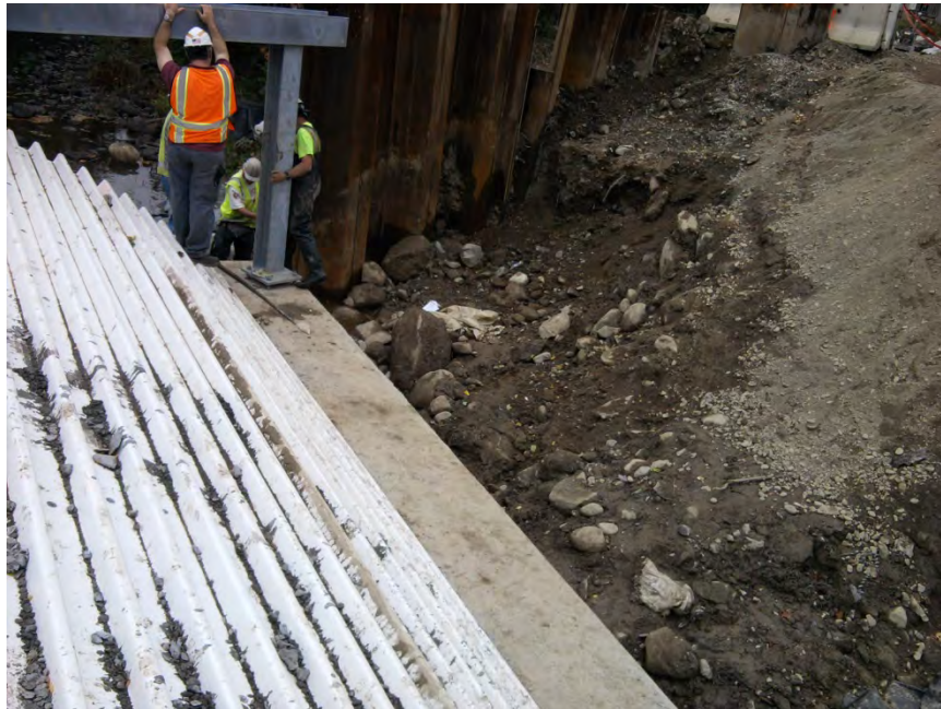
Figure 4: Headwall frame construction at Jenkins Bridge
