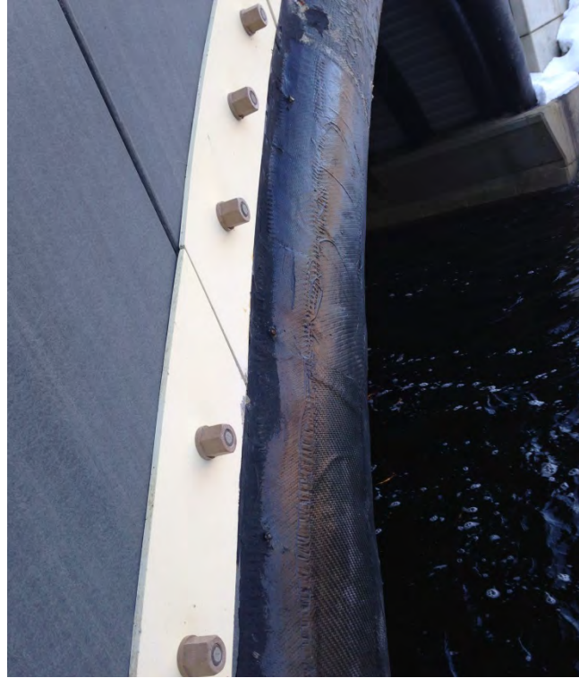
Figure 37 - Close up View of Repair on Upstream Tube (2014)
