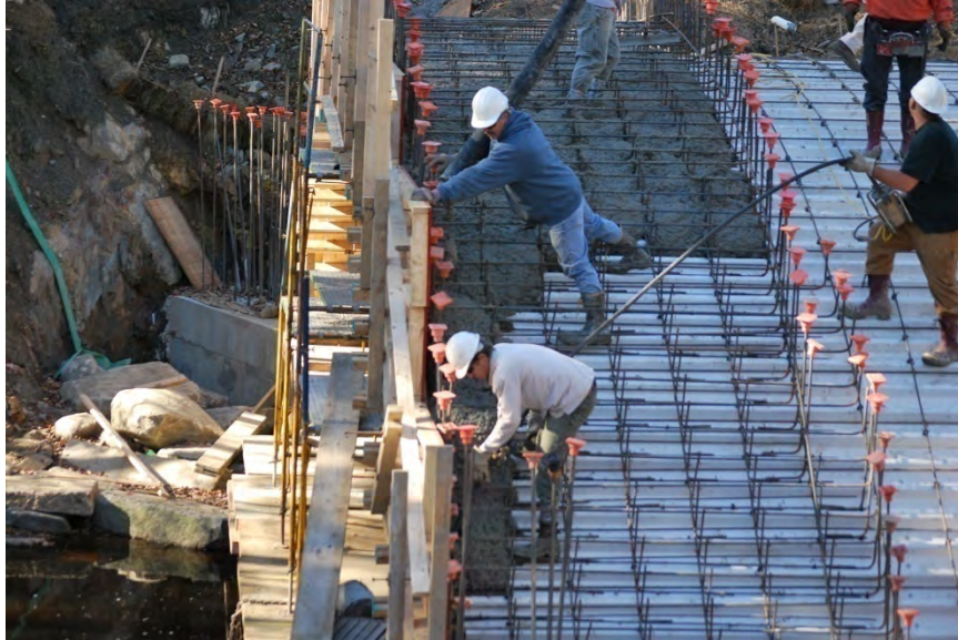
Figure 1: Concrete placement at base of headwall (Perkins Bridge)
