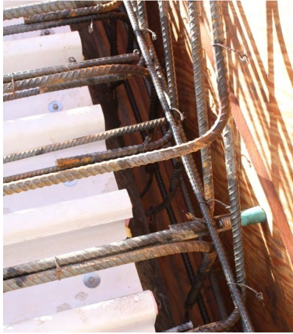
Figure 3: Details of rebar at base of headwall
