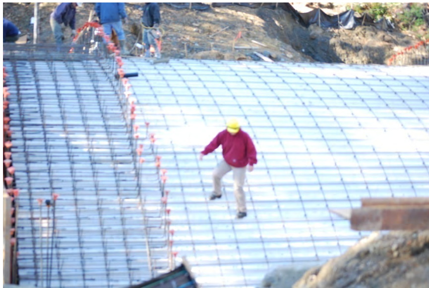
Figure 2: Rebar mat allowed for walking during construction
