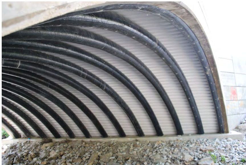
Figure 29: Underside of bridge
