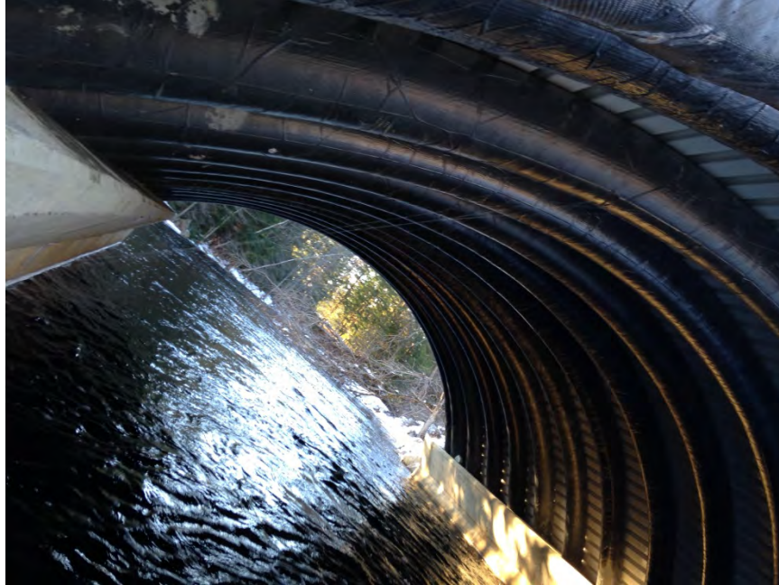
Figure 38 – Underside of Jenkins Bridge (2014)
