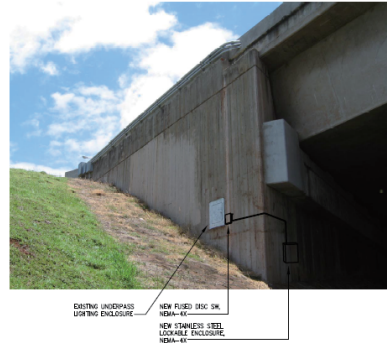
(b) Equipment elevation
