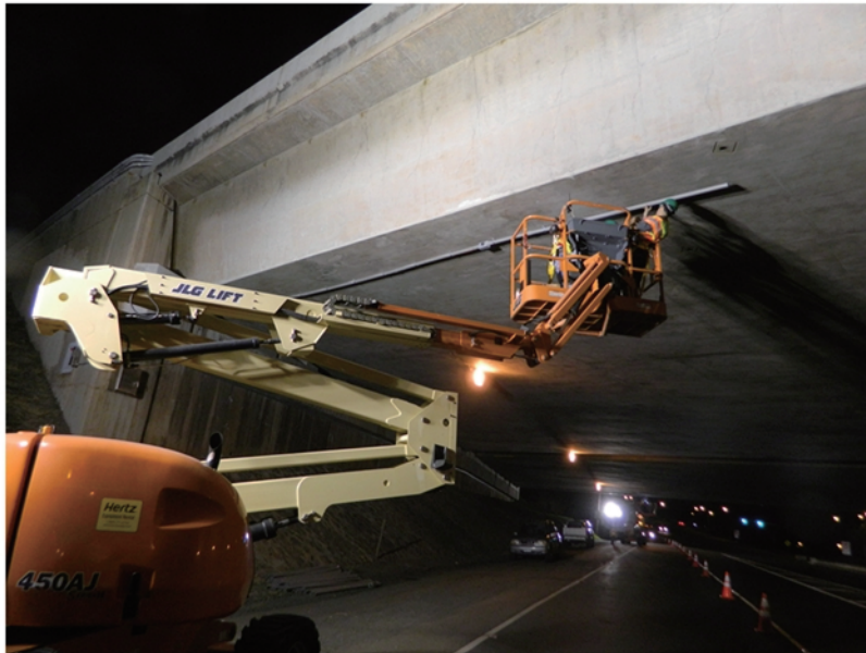
Figure 5.17: Conduit installation
