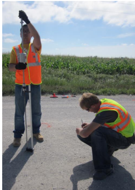
Figure 11. Dynamic cone penetrometer (DCP) test
