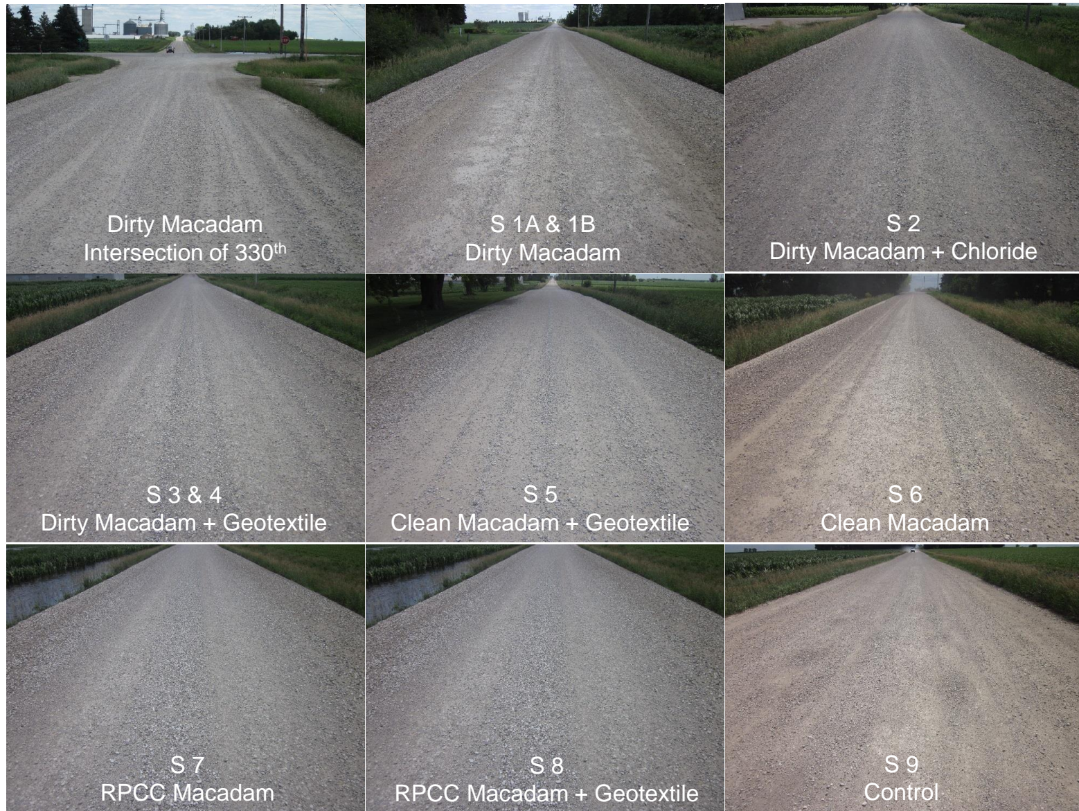
Figure 128. Survey photos of Vail Avenue demonstration sections (July 3, 2014)
