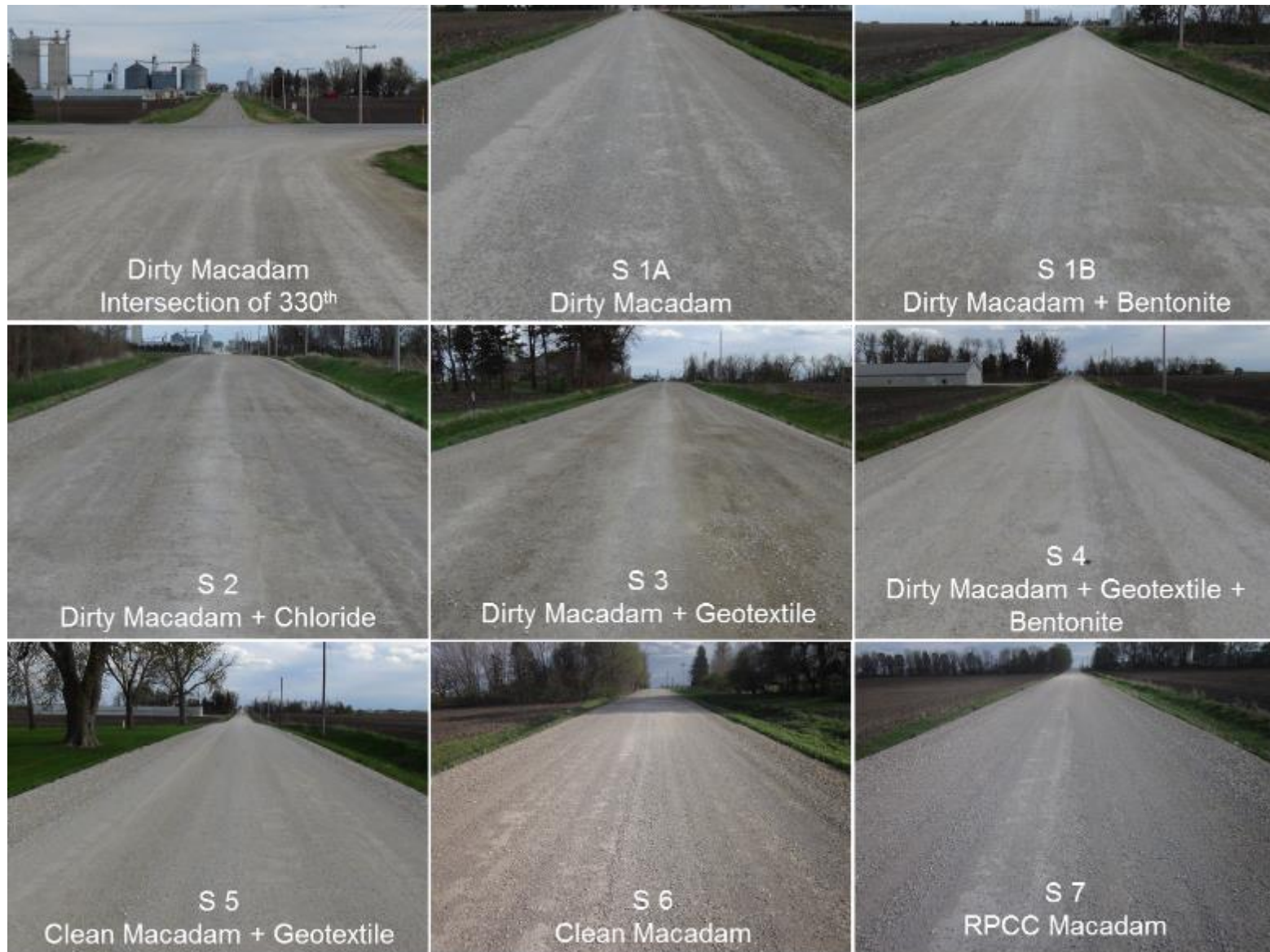
Figure 133. Survey photos of Vail Avenue demonstration sections (April 21, 2015)
