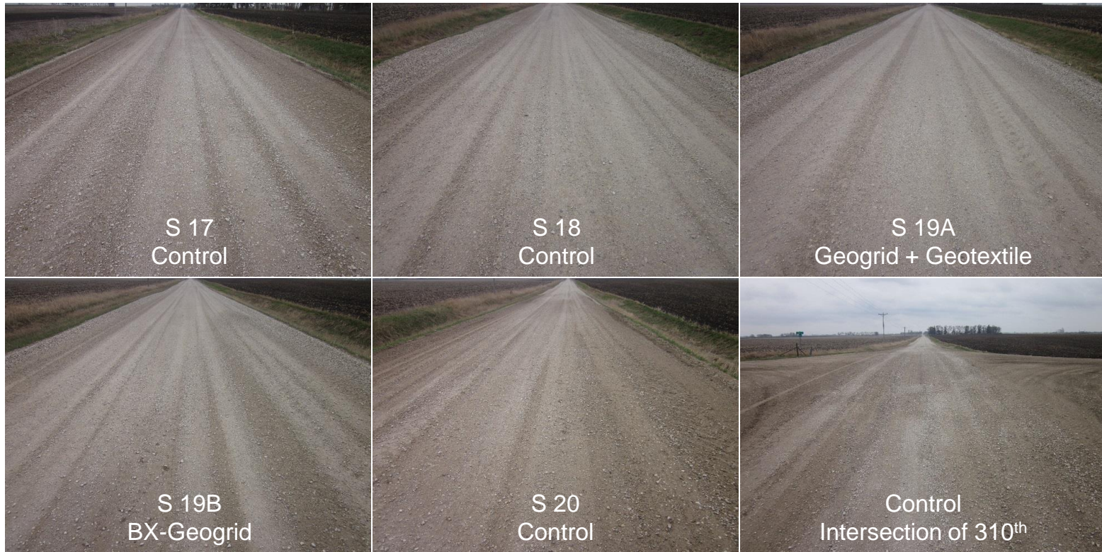
Figure 125. (continued). Survey photos of Vail Avenue demonstration sections (April 21, 2014)
