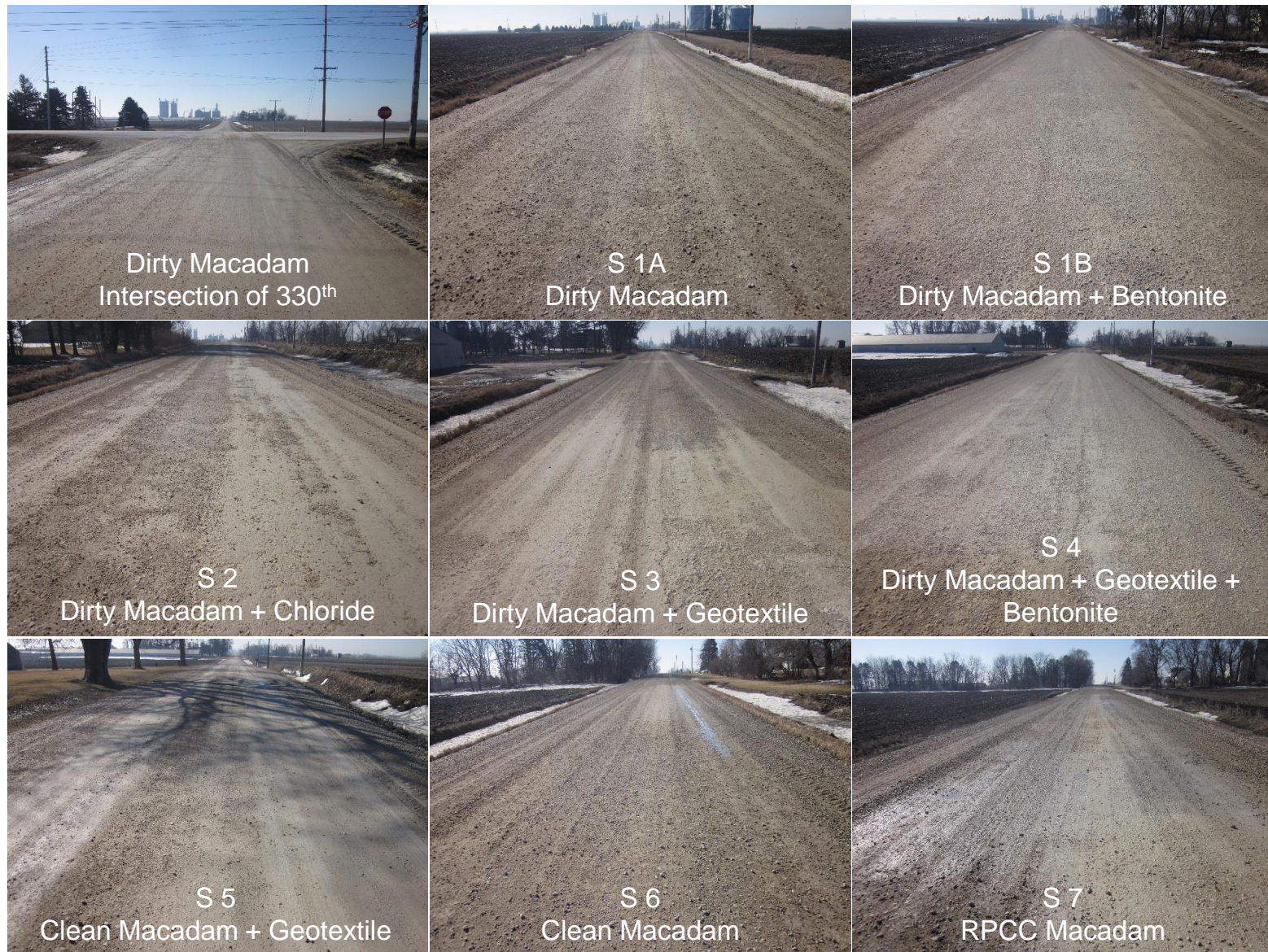
Figure 132. Survey photos of Vail Avenue demonstration sections (March 10, 2015)
