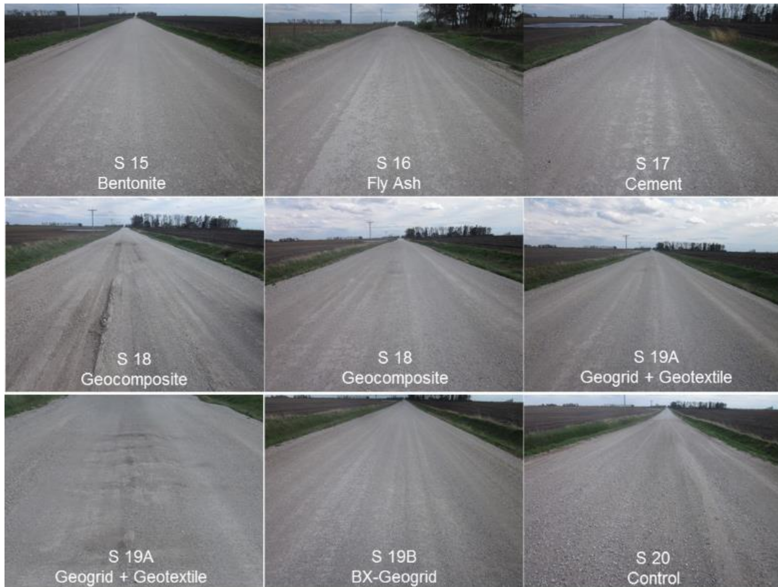
Figure 133. (continued). Survey photos of Vail Avenue demonstration sections (April 21, 2015)
