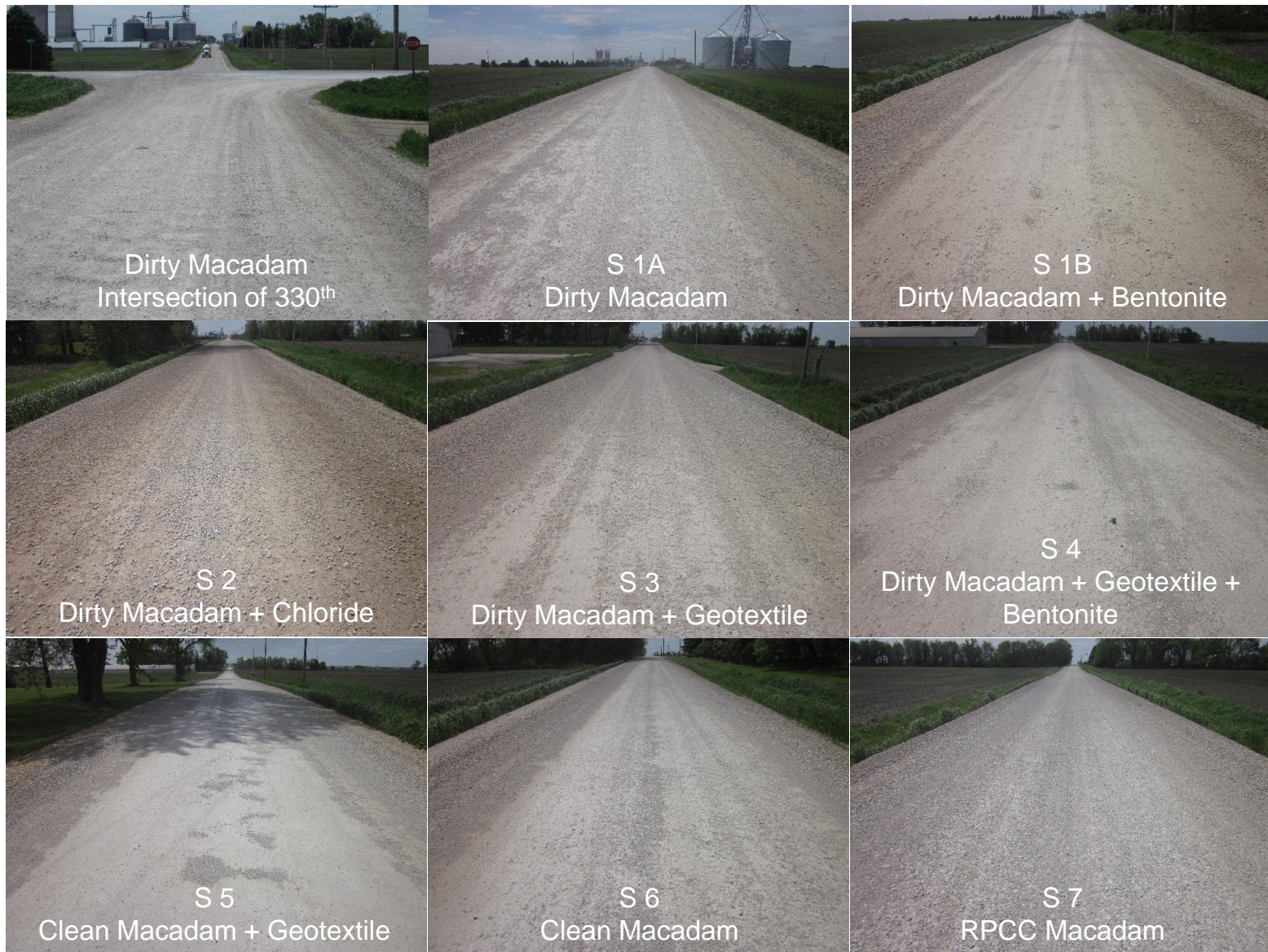
Figure 134. Survey photos of Vail Avenue demonstration sections (May 19, 2015)
