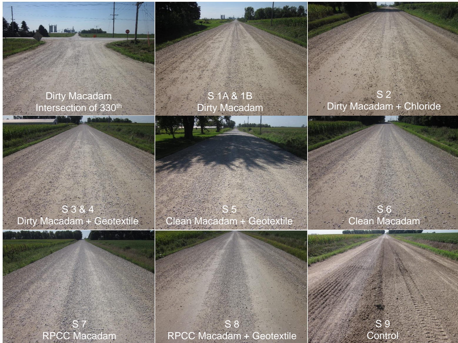
Figure 129. Survey photos of Vail Avenue demonstration sections (September 2, 2014)
