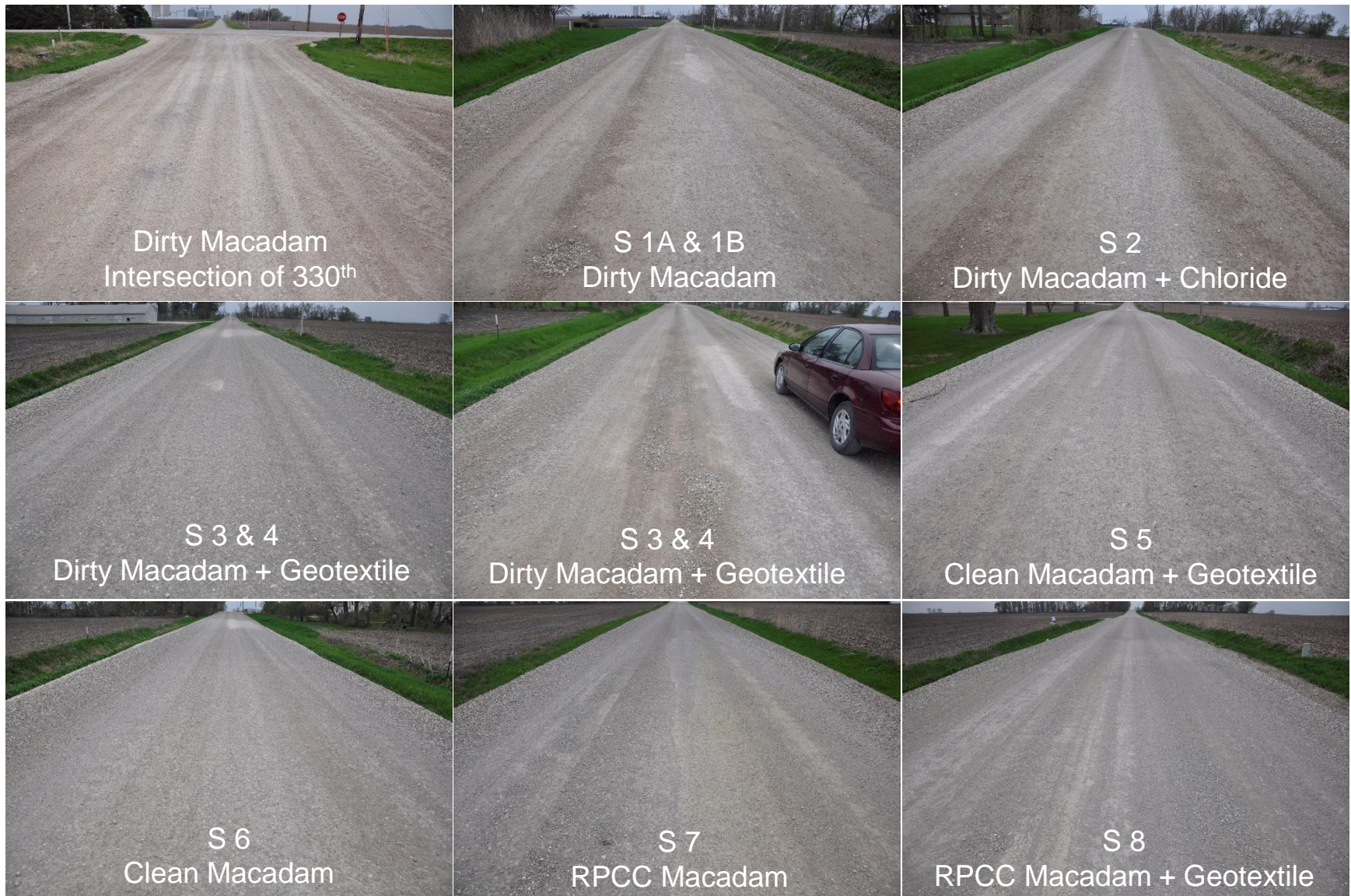
Figure 126. Survey photos of Vail Avenue demonstration sections (May 8, 2014)
