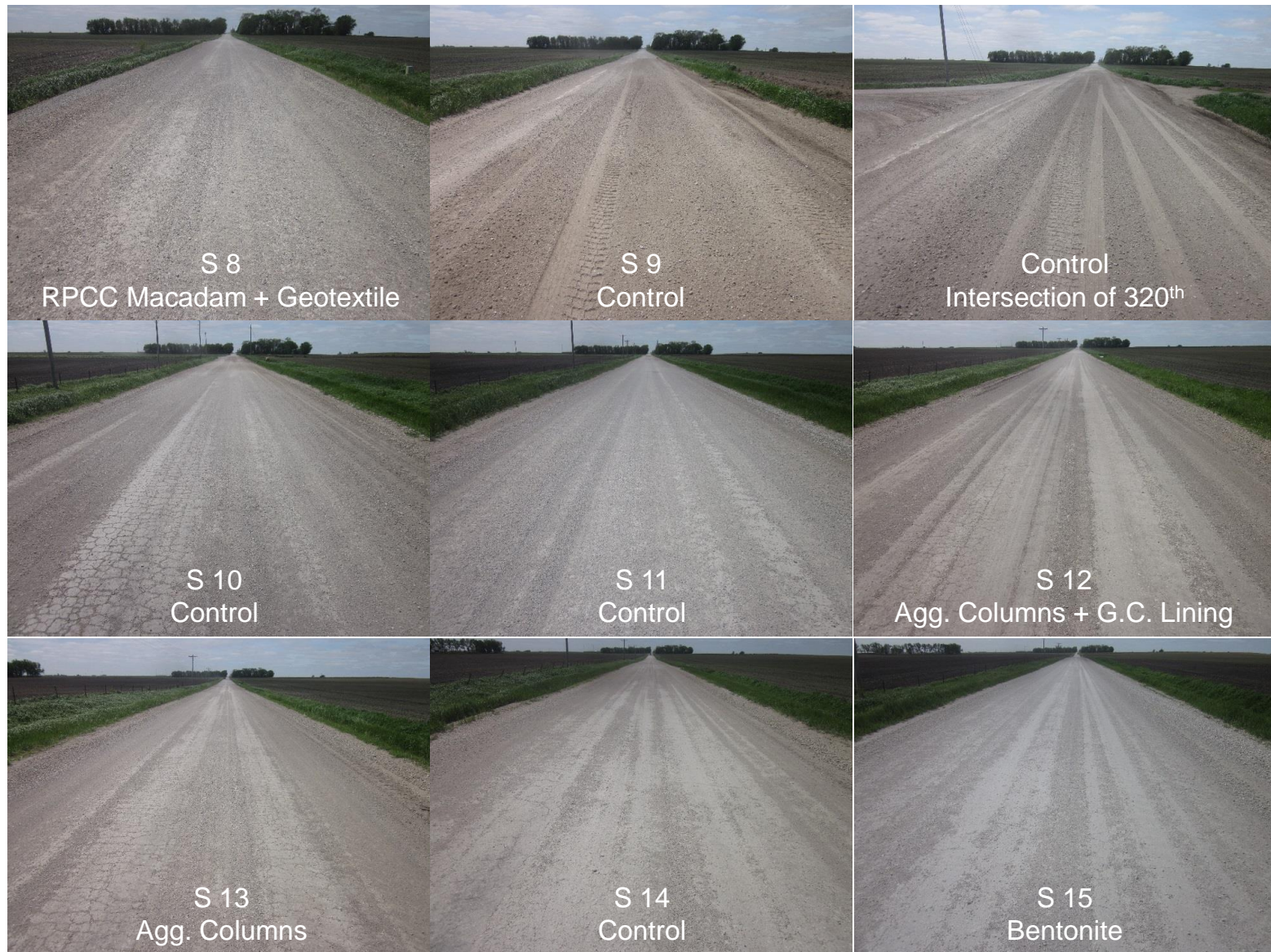
Figure 134. (continued). Survey photos of Vail Avenue demonstration sections (May 19, 2015)
