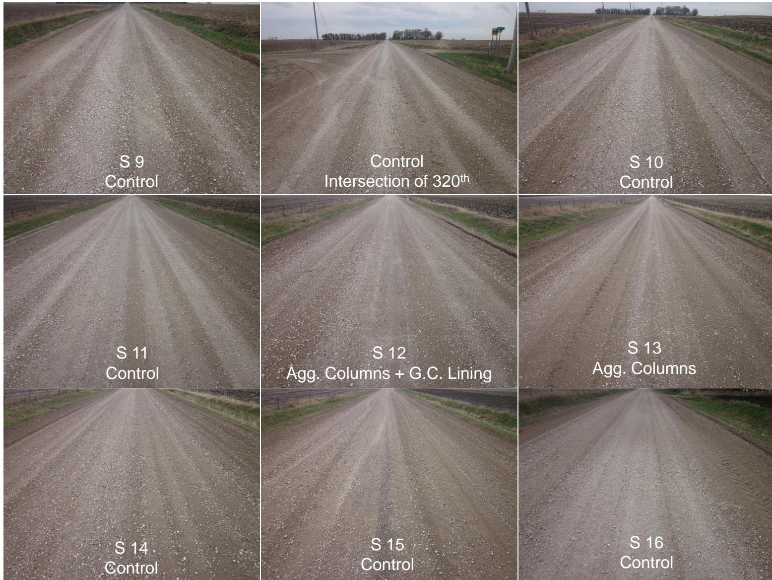
Figure 125. (continued). Survey photos of Vail Avenue demonstration sections (April 21, 2014)
