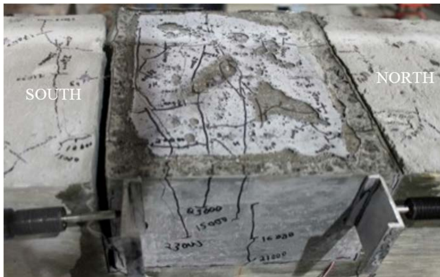
Figure 33. UHPC Pocket in Specimen U-4-5-II After Failure Showing South Interface Separation
