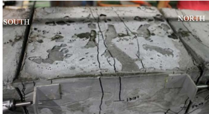
Figure 30. UHPC Pocket in Specimen U-4-5-I-E Showing Interface Separation and Flexural Cracks
