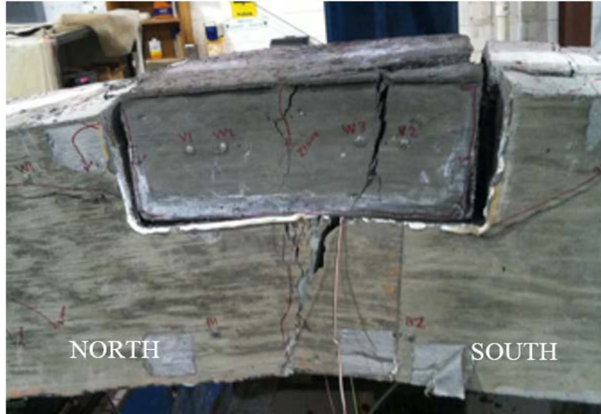
Figure 36. VHPc Pocket in Specimen V-4-6-I Showing Interface Separation and Splitting Cracks
