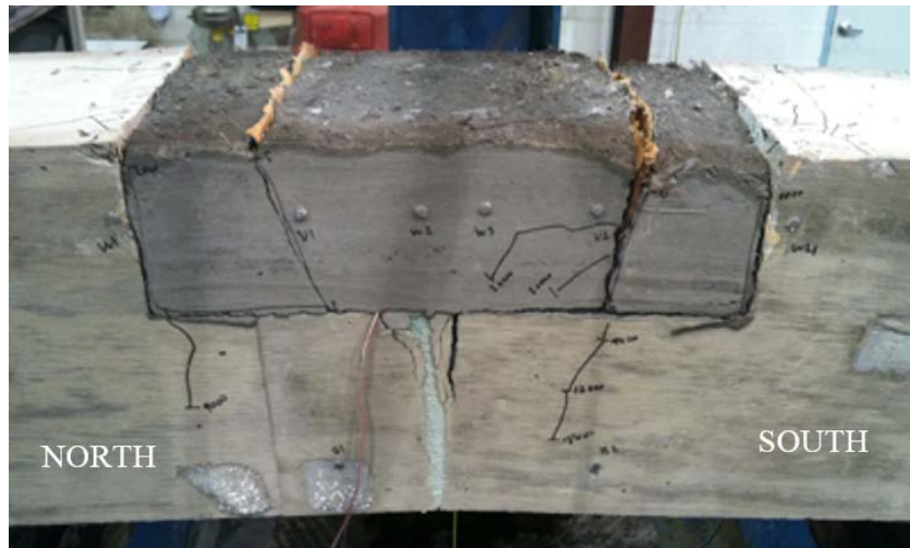
Figure 40. VHPC Pocket in Specimen V-4-3-I at End of Load Application Showing Interface Separation
