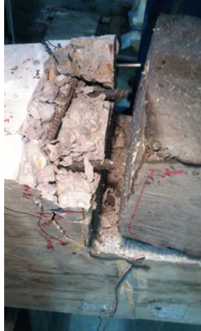
Figure 38. Specimen V-4-5-II at End of Load Application Showing the Reinforcing Bars Ruptured
