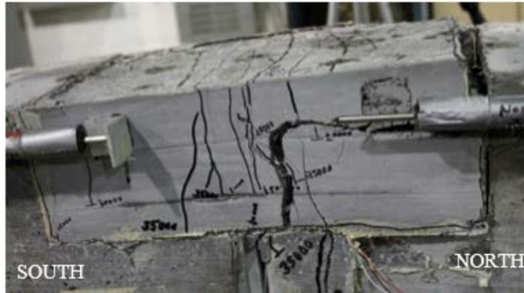
Figure 51. Side View of UHPC Pocket in Specimen U-6-6-I-E After Failure Showing the Effect of Prying Action
