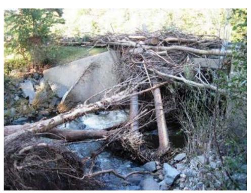
(b) Wilmington VT100-B53 Bridge: obstructions at a small single span resulting in blockage and overtopping
