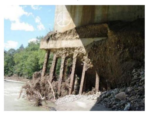
(b) Dummerston VT30-B9 Bridge: scour beneath the concrete spread footing, with settlement resulting in the cracking of the foundation.
