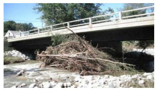
$(a) \ \ Walling for d\ VT 140-B 10\ Bridge:\ debris\ build up\ on\ a\ pier,\ reducing\ the\ flow\ area$
