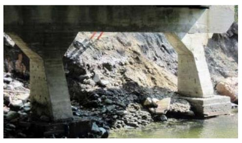
(a) Halifax C2001-B17 Bridge: loss of original riprap and backfill, resulting in the free standing abutments and scour to beneath the footing of the spread footing base
