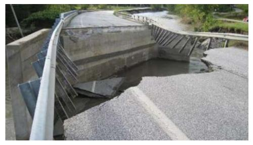
(a) Braintree VT112A-B6 Bridge: erosion behind the wing-walled abutment, with complete loss of the bridge approach
