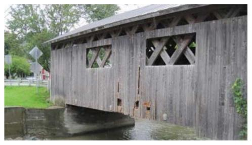
(a) Montgomery C2001-B5 Bridge: damage to the sideboards of a covered bridge
