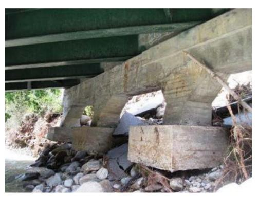
(b) Jamaica VT30-B78 Bridge: flanking behind the wingwall abutment, with scour beneath the bridge foundation, with no apparent damage to the concrete foundation, and no major settlements to the foundation
