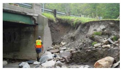
(a) Wardsboro VT100-B68 Bridge: flanking erosion behind the abutment, and minor scour to the footing
