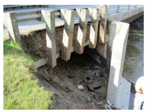
$(b) \ \ Jamaica\ VT30-B40\ Bridge: flanking\ behind\ the\ abutment\ undermining\ the$   $approach\ slab$
