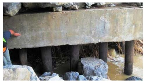
(a) Clarendon US7-B96 Bridge: scour beneath the foundation, exposing several feet of wooden piles
