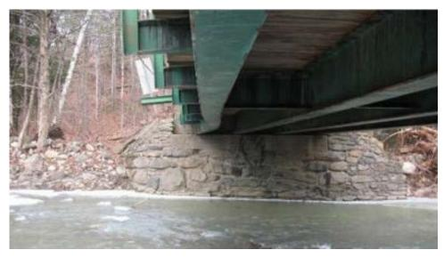
(b) Marlboro C3014-B23 Bridge: damage to the main beam of the bridge from debris impact
