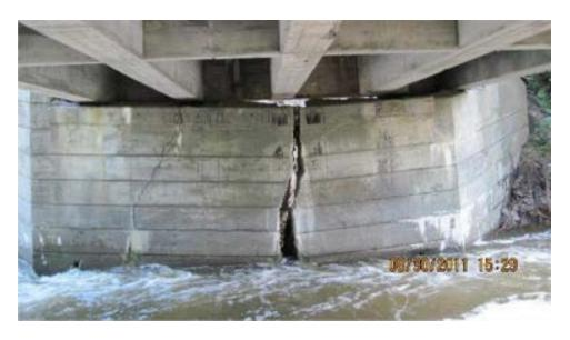
(a) Brownington C2001-B9 Bridge: fracture to the foundation, due to scour beneath the footing and settlement of substructure
