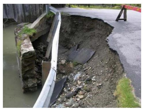
(b) Warren FAS188-B6 Bridge: Channel erosion and flanking behind the wingwall, with scour hole at the toe
