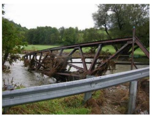
(b) Moretown C3024-41 Bridge: collapse of the steel truss bridge from the apparent loss of one of the bridge foundations
