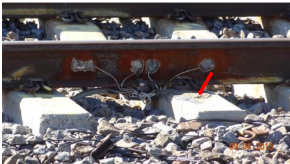
Figure 1. Photograph showing strain gages on rail and LVDT location on tie (see arrow)
