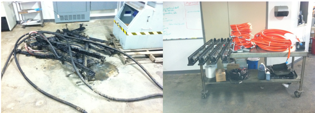
Figure 13: Used components were removed (left) and new components provided by OEM 1 were installed on the cleaned out lubricators
