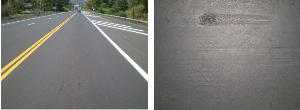
Figure 6 – Flushing Located on Rt 20 in Morrisville, NY
