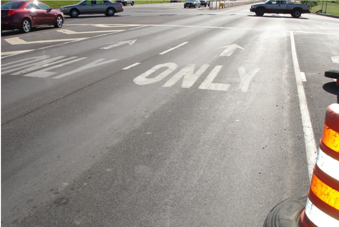
Figure 7 – Flushing at Intersection on Rt 5
