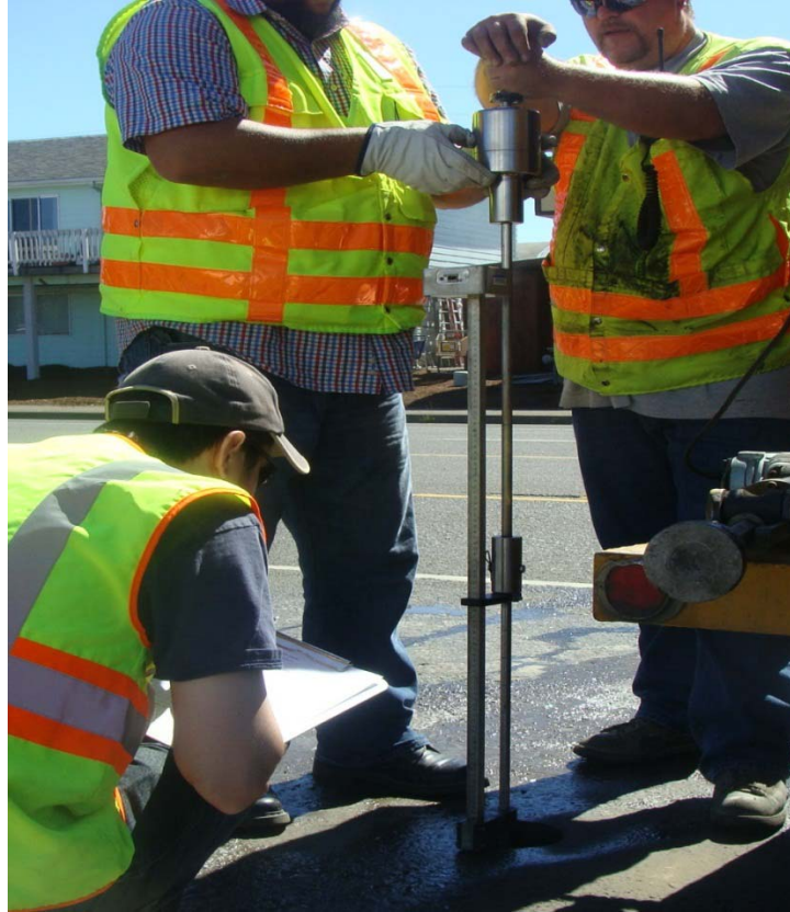
Figure 4.8: Photos of Dynamic Cone Penetrometer Testing
