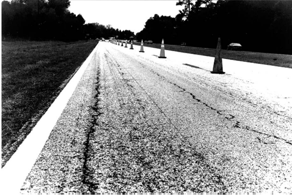
Figure 2.1: Lane Exhibiting Surface Initiated Top-Down Cracking in Both Wheelpaths (Myers et al. 2001)
