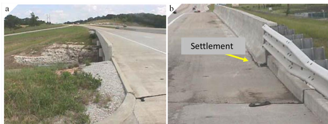
Figure 2(a) No settlement on bridge approach slab with unused mudjack holes shown, and (b) Differential settlement occurred on a bridge approach slab (Petry et al., 2002)
