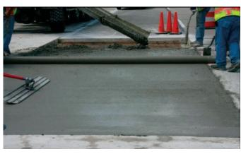
New rapid set mixtures are showing user-friendly characteristics, good potential for durability and OTT times within six hours of batching.
