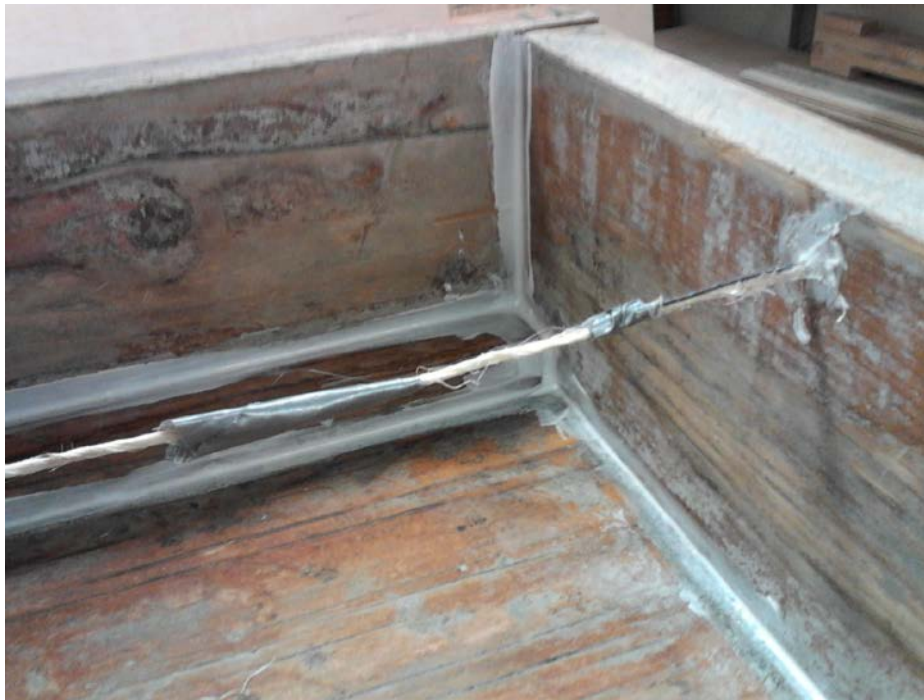
Figure 4.2: Thermocouple Wire Setup Within Slab Forms
