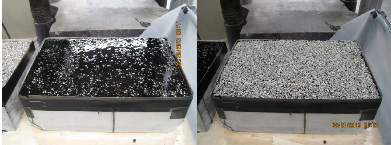
Figure 4.17: Placement of Course Two of Epoxy (left) and Aggregate (right)
