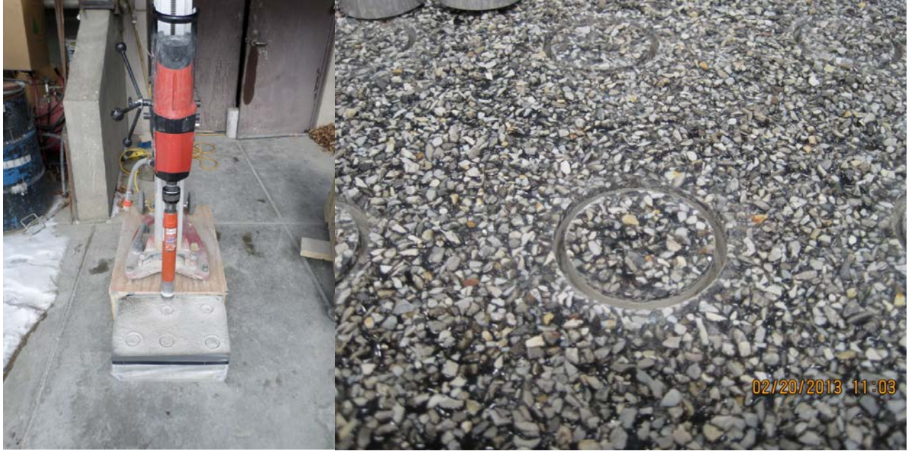
Figure 4.18: Coring Setup (left) and a Core Through the Overlay into the Concrete (right)
