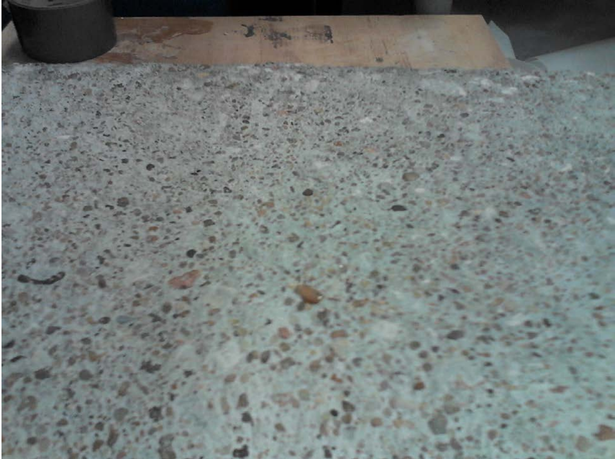
Figure 4.14: Close Up of Concrete Surface After Sandblasting
