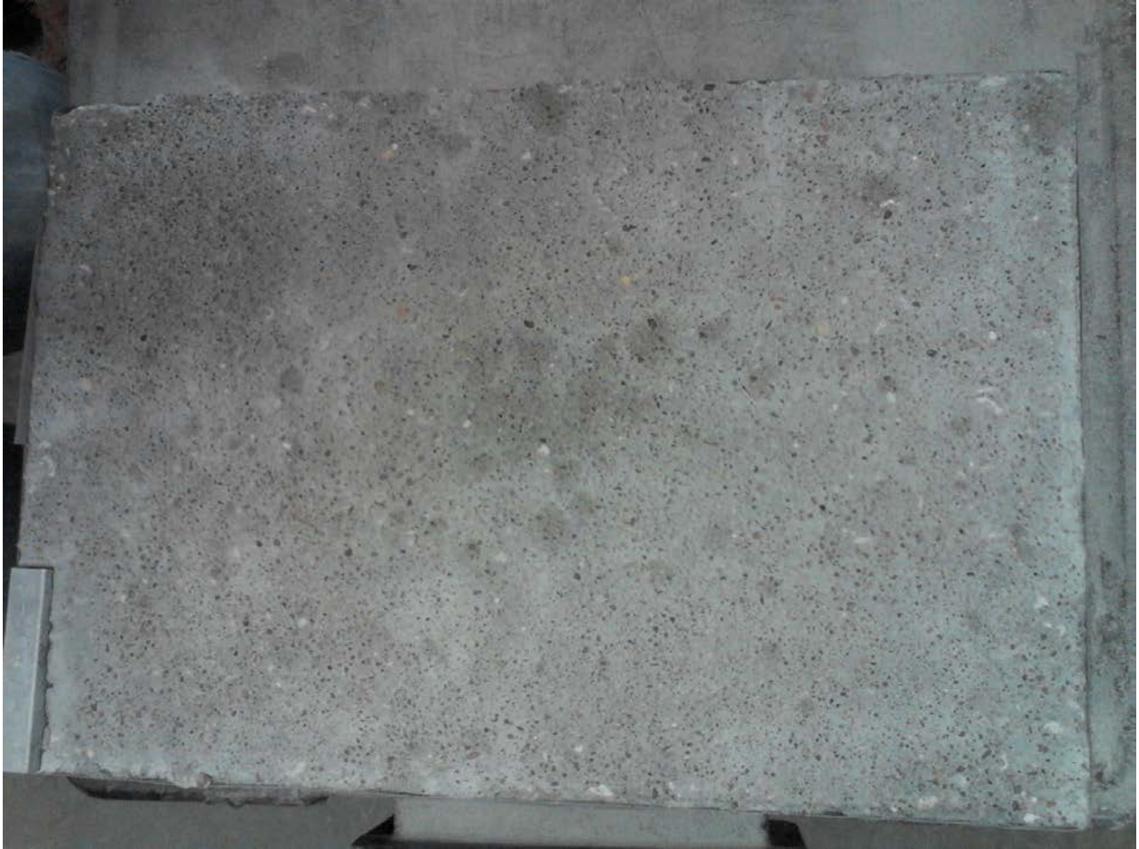
Figure 4.13: Sandblasted Surface with Visible Large Aggregates
