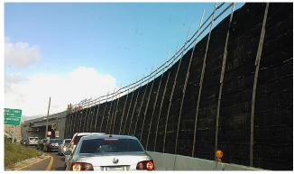
*The black wall (right) is an earthwork, retained by geotextile, which supports a section of I-295 under construction.*
