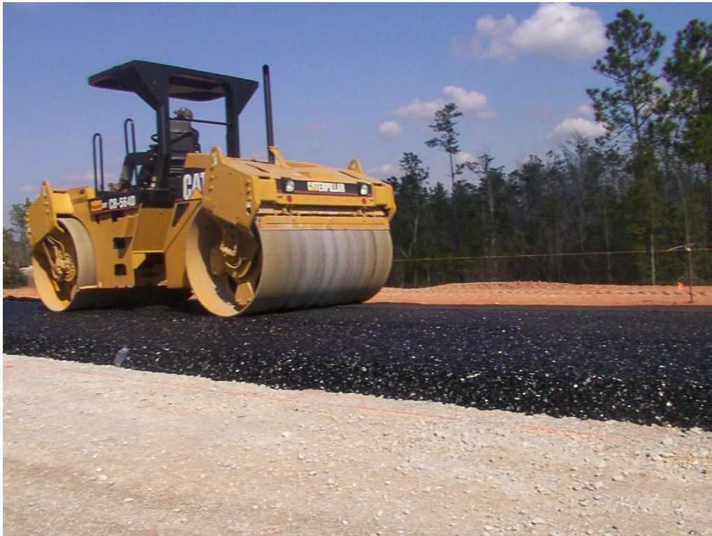
Figure 2: ADC Under Construction for Mini-Experiment
