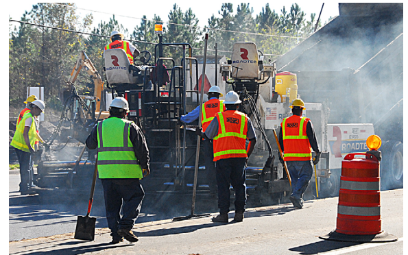
The durability of asphalt mixes for Florida roads is improved by the use of modifiers.
