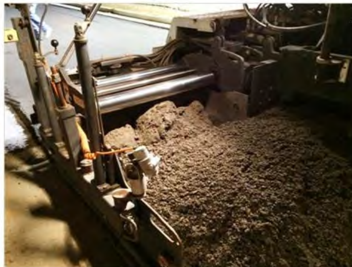
Figure 13. Hardened RCC in Paver
