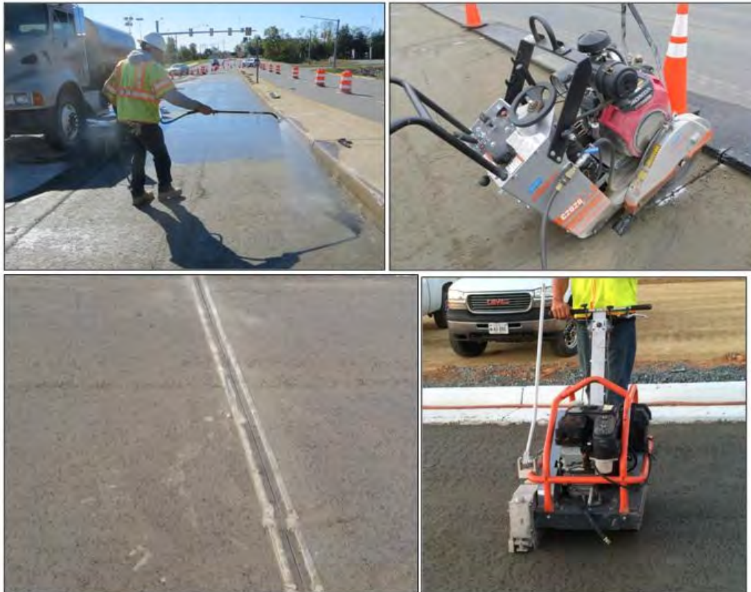
Figure 14. Water Curing and Saw Cutting of Joints
