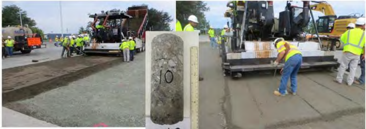
Figure 5. First Trial Installation of RCC
