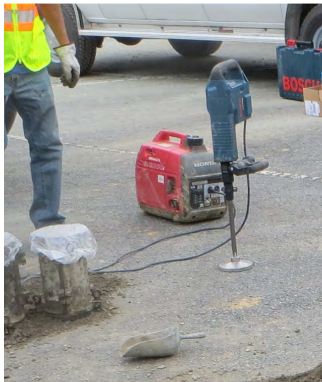
Figure 1. Vibrating Hammer to Prepare RCC Cylinders
