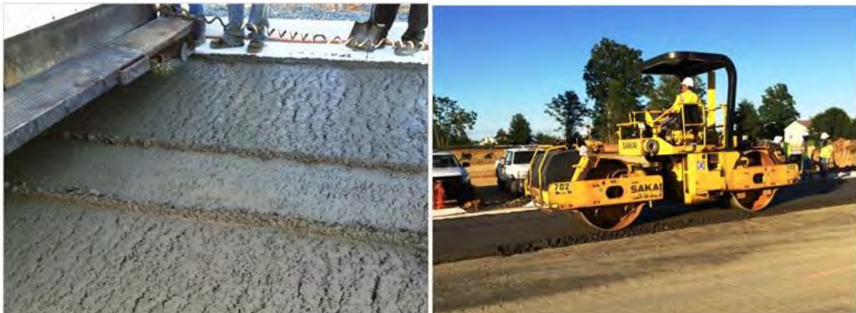
Figure 10. Settlement of RCC Attributable to Wet Mixture
