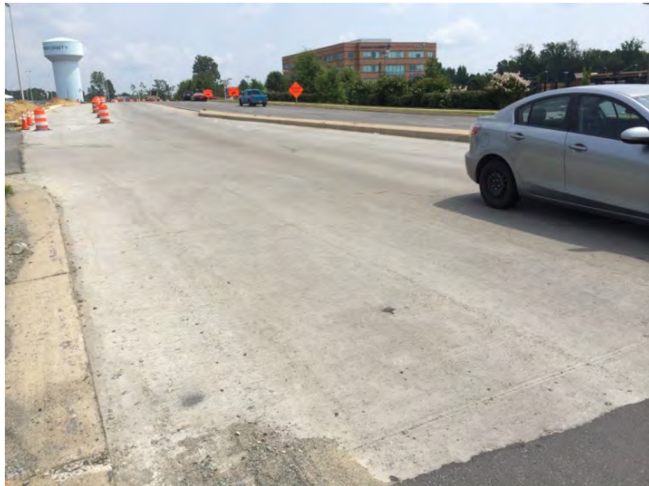
Figure 15. Completed RCC on Staffordboro Boulevard
