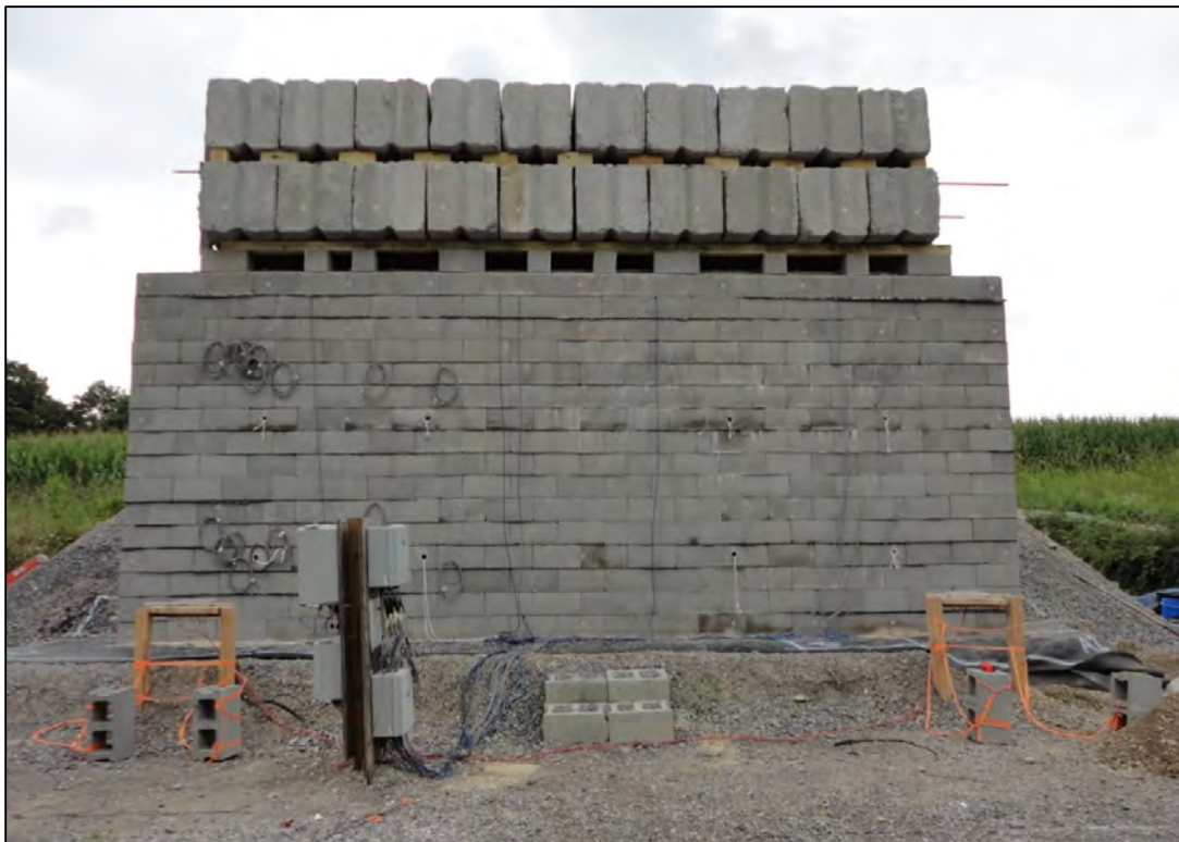
Figure 25. Front View of Abutment Before Testing, RSF Removed Around Region A1
