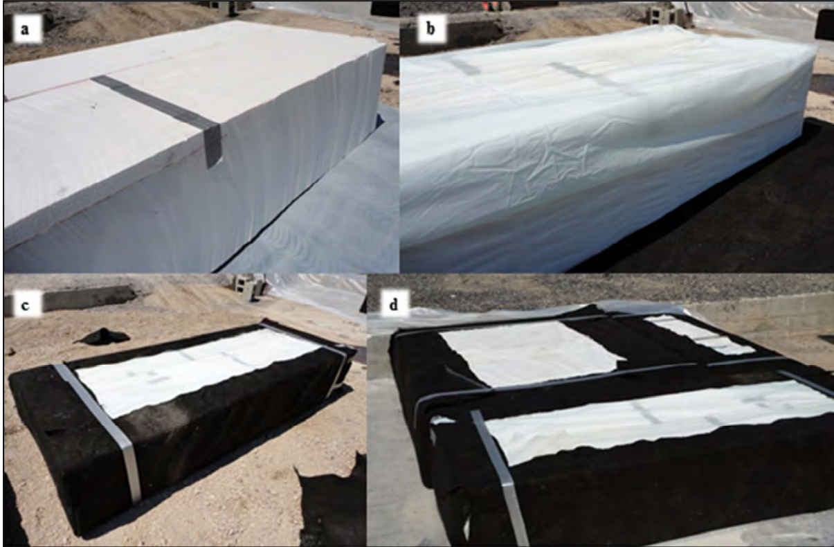
Figure 8. (a) Placing Geofoam on Top of Geonet and Plastic; (b) Wrapping Geofoam in Plastic; (c) Wrapping Geofoam and Plastic in Non-Woven Geotextile; (d) Arranging Packaged Geofoam in Testing Configuration
