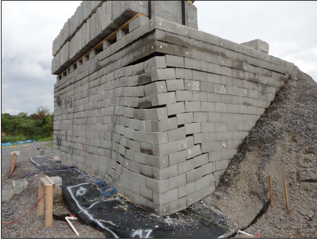
Figure 29. Corner a of Abutment After Test A2
