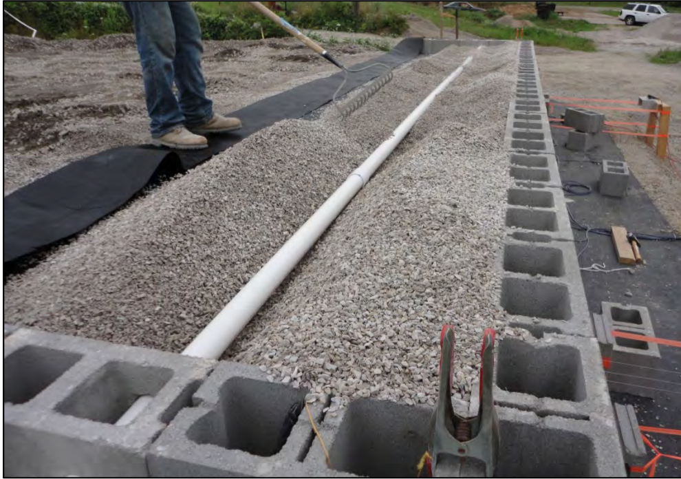
Figure 21. Example of Settlement Profiling Tube
