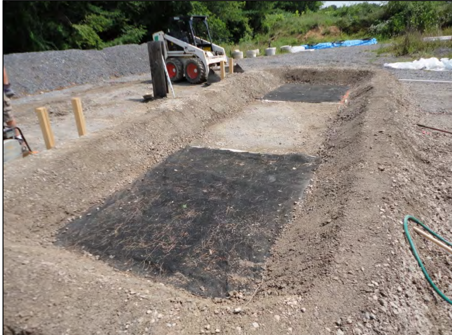
Figure 10. Berm to Construct RSF
