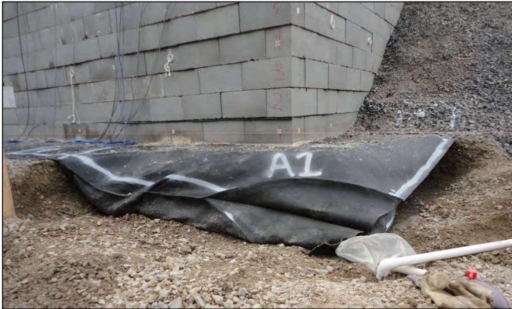
Figure 24. RSF Berm Removed for Test A1
