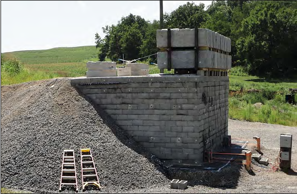
Figure 15. Completed Abutment
