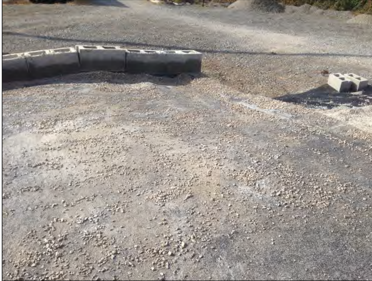
Figure 80. Side A, Level 5 During Deconstruction
