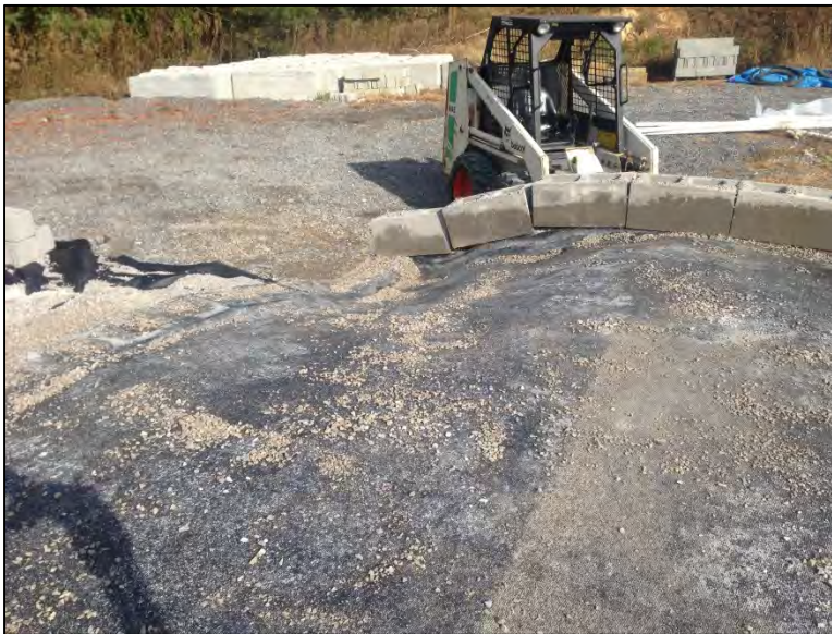
Figure 81. Side B, Level 5 During Deconstruction
