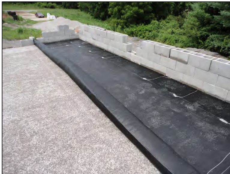
Figure A-23. Installing Geotextile Fabric With Attached Strain Gages
