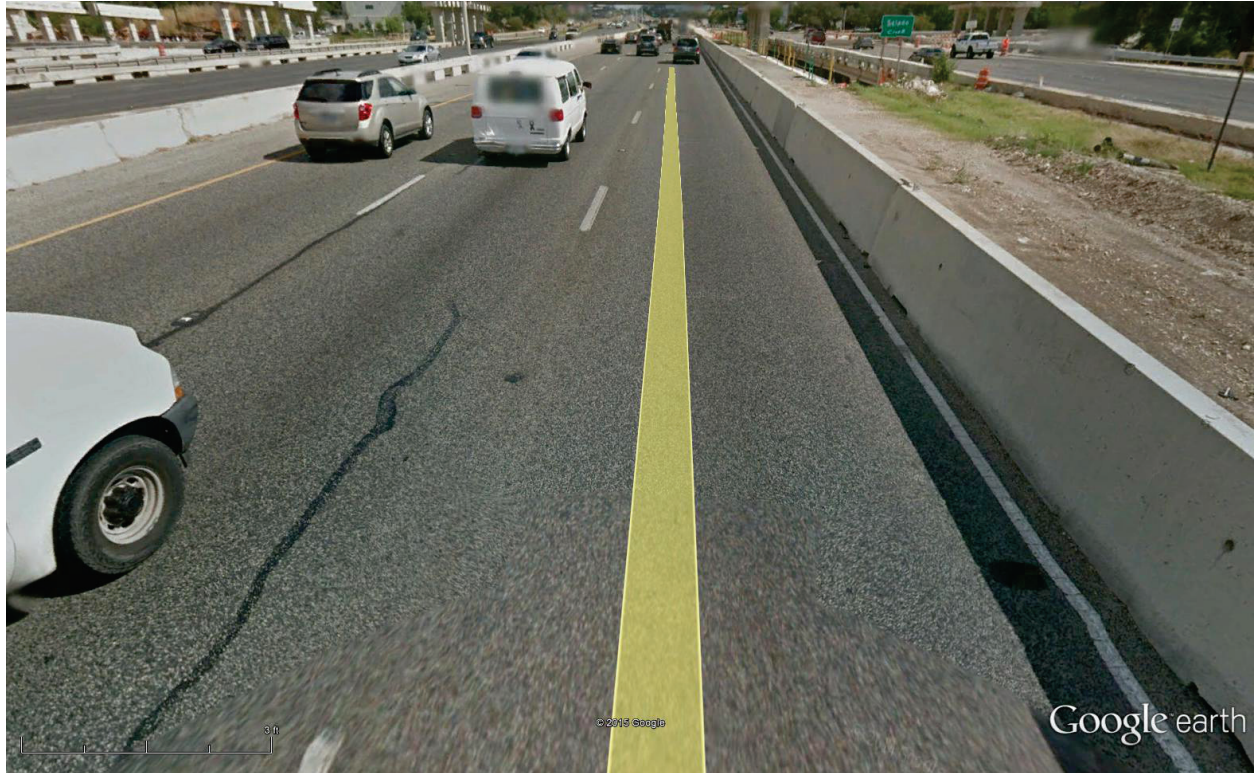
Figure 19. Street View of Site with Narrowest Right Shoulder Width.
