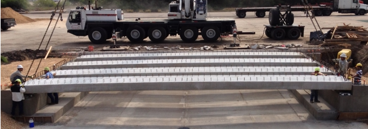
(a) Slab Beam Placement
