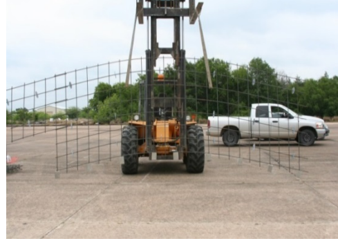
(b) Rebar Mesh Installation
