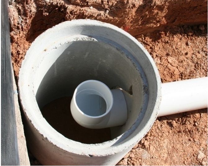
(b) Manhole Placement
