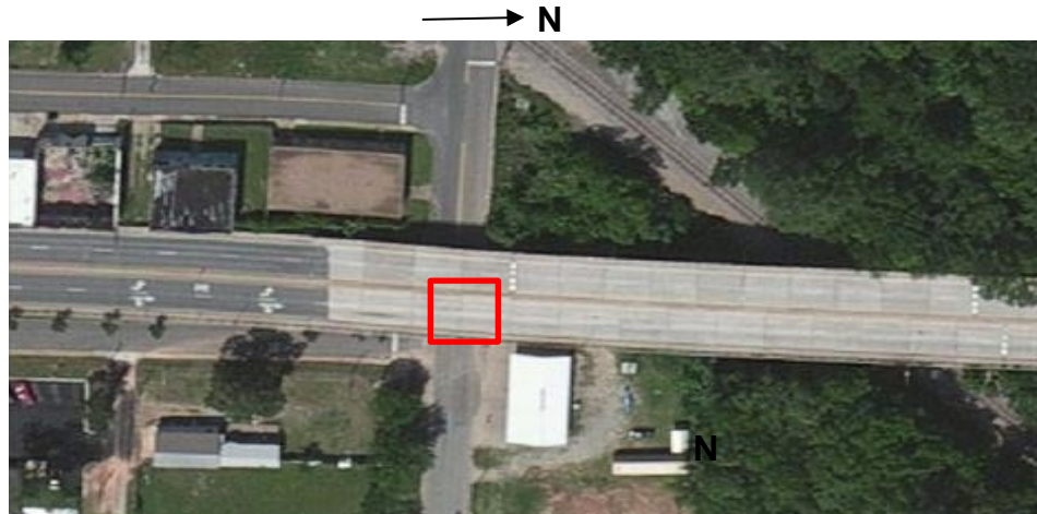
(a) Location of US 69 Bridge over Day Street (Google Maps 2005)
