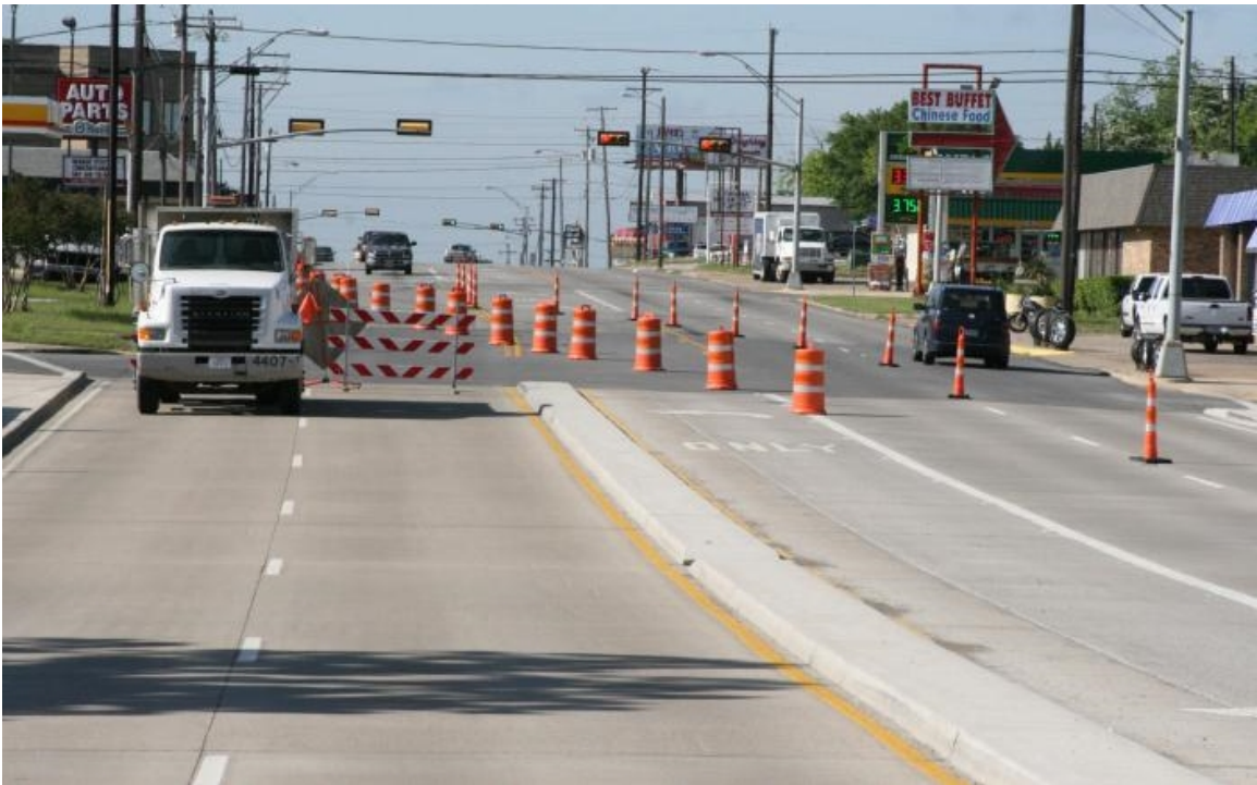
(b) Traffic Control on US 69 (Looking South from Bridge)
