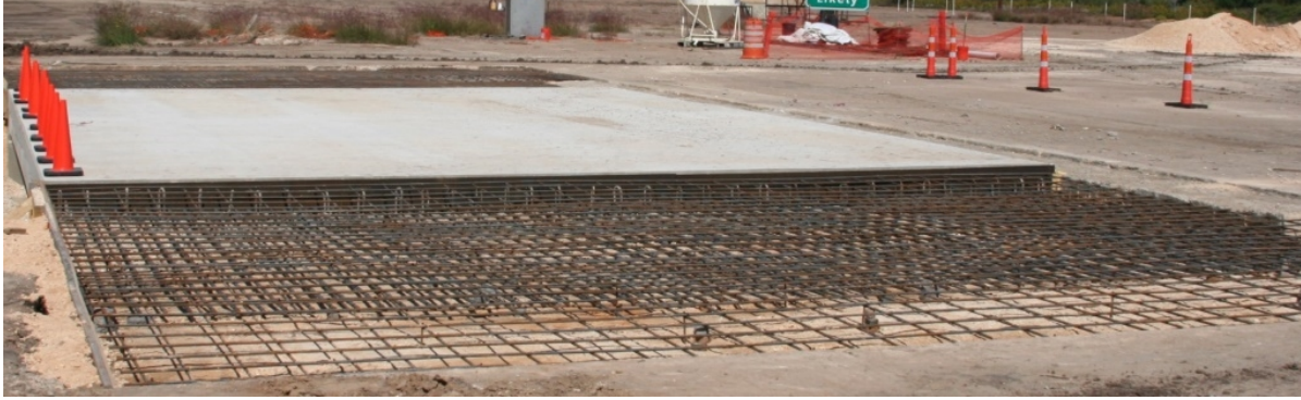
(b) Approach Slab Reinforcing Mesh
