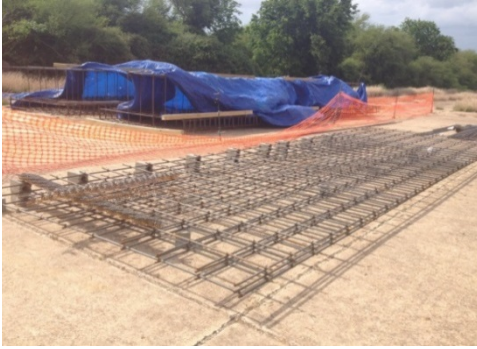
(a) Rebar Tying
