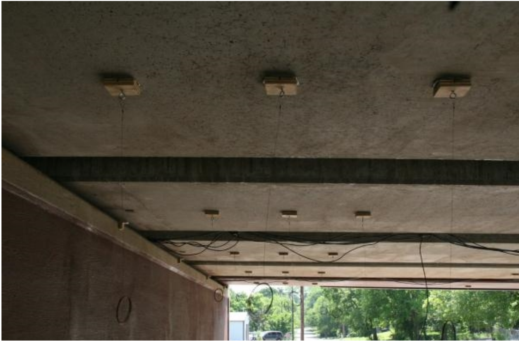
(b) LVDT and String Potentiometer Setup Installation
