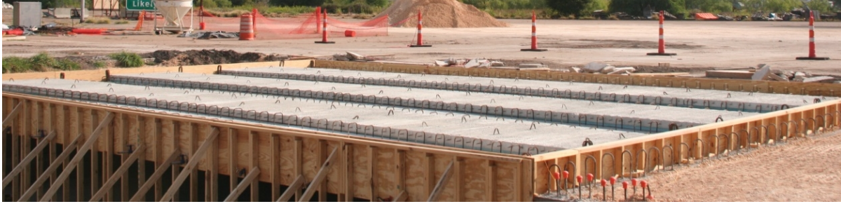
(a) Deck Formwork Construction
