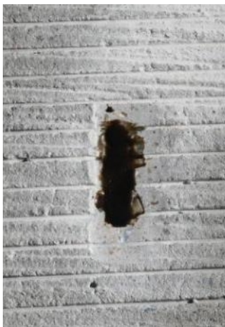
(c) Top Surface Preparation
