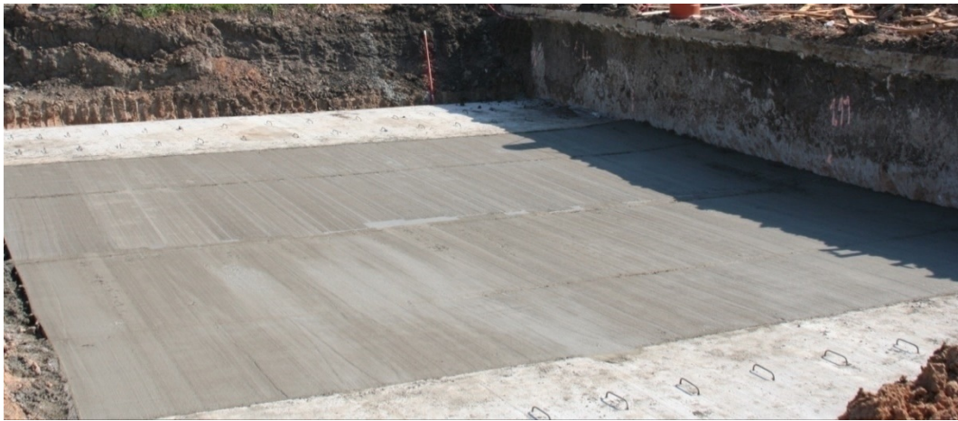
(c) View of Slab-on-Grade after Broom Finish
