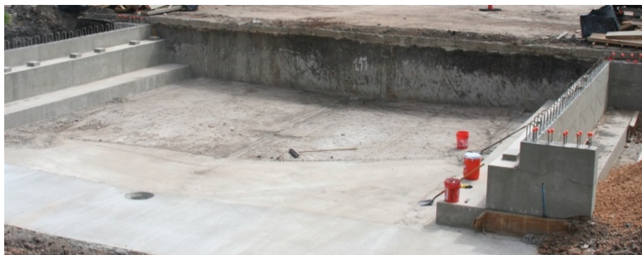
(b) View of the Substructure after Removal of the Forms
