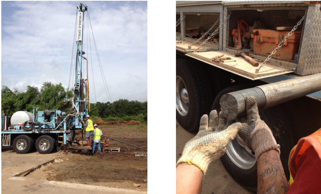
Figure B.2. Soil Testing of the Bridge Site.
