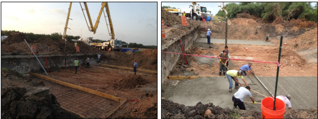
Figure B.9. Reinforcing Bar Mesh for the Slab-on-Grade.
