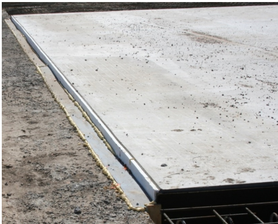
(a) Expansion Joint and Steel Sheet Form.
