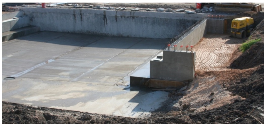
(c) Backfilling and Compaction Process
