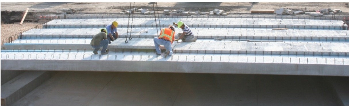
(c) Placement of Precast Concrete Panels
