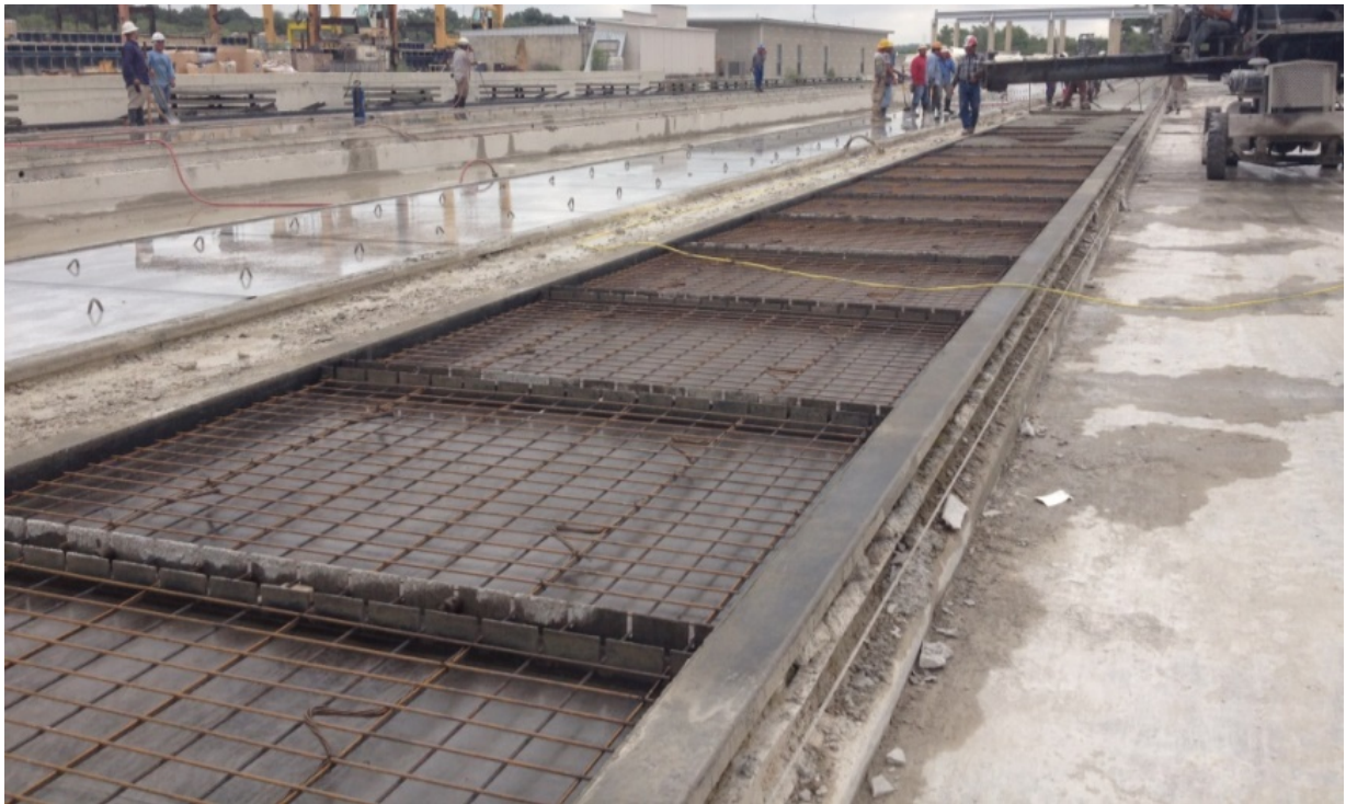
Figure B.18. Precast Concrete Panel Construction.
