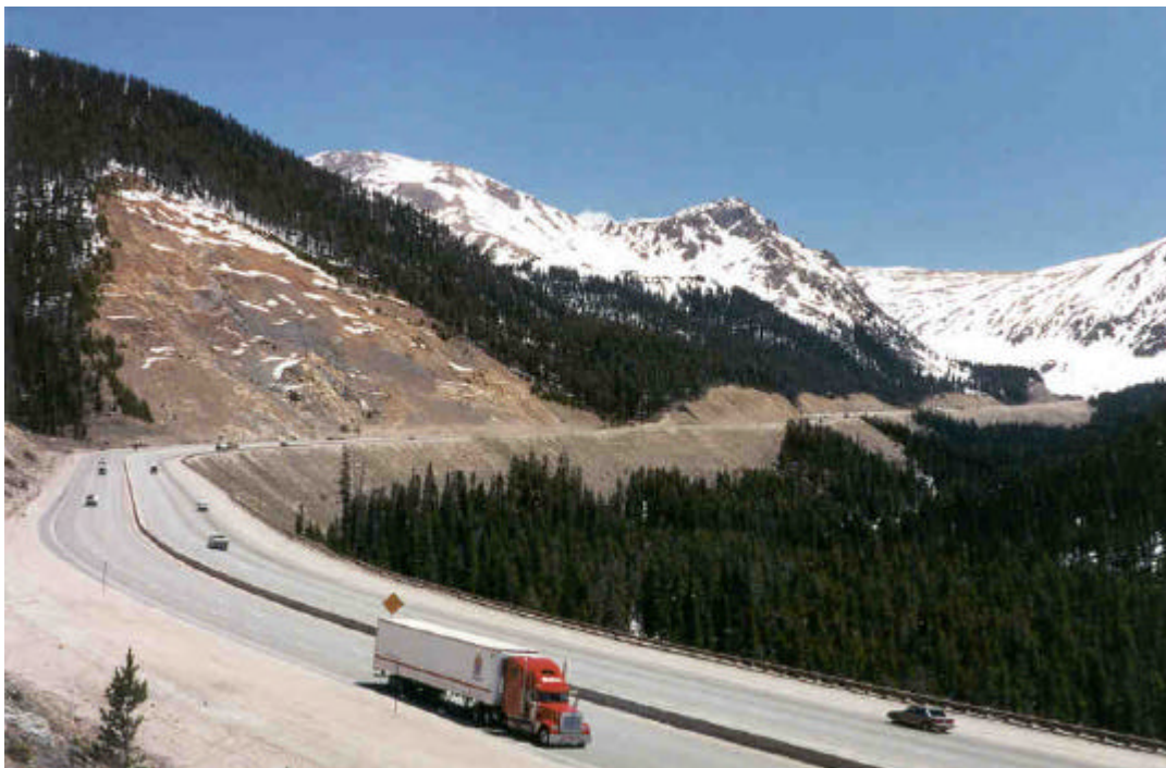
Figure 8: Photo of I-70 Two Miles West of Eisenhower Tunnel
