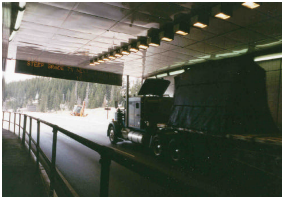
Figure 6: Photo of Speed Warning Message Display in Eisenhower Tunnel
