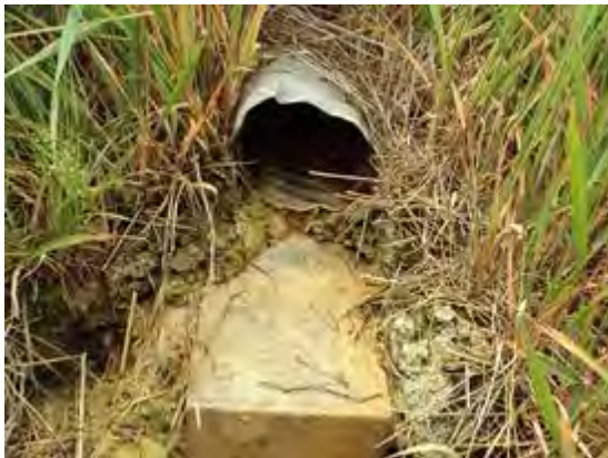
Good drainage pad installation
