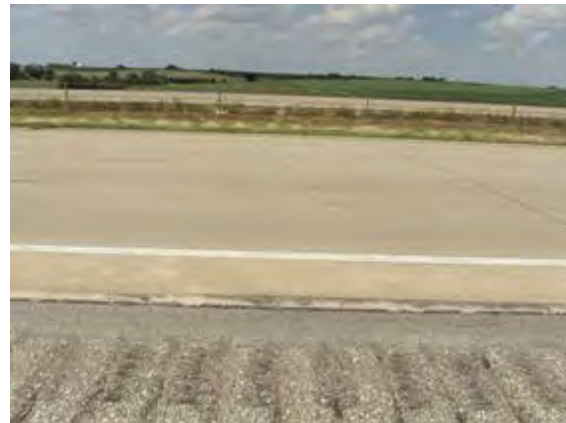
No pavement surface distress
