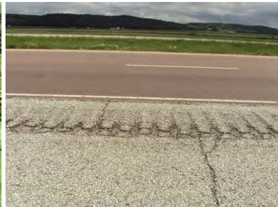
Transverse cracking
