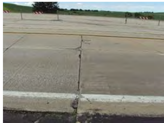
Corner cracking
