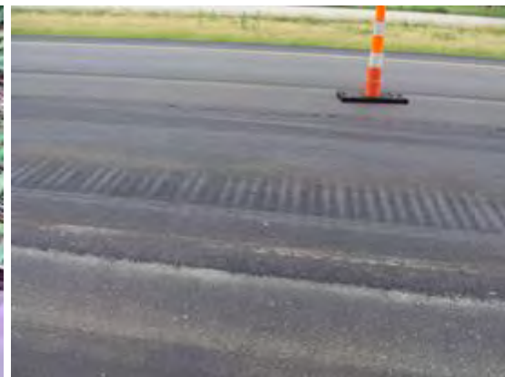
New HMA overlay
