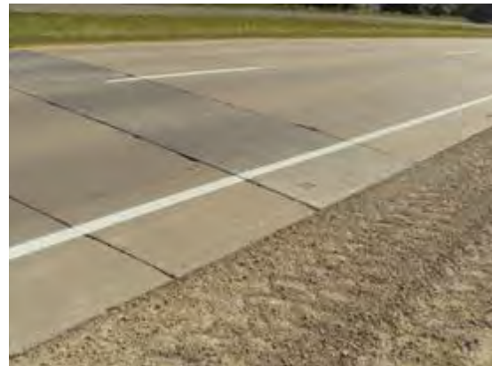
Pavement patching due to culvert
