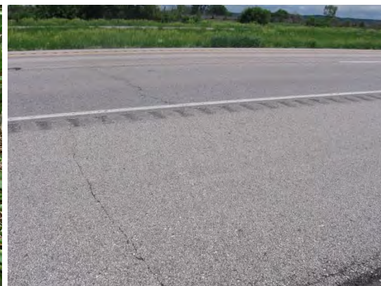
Transverse cracking
