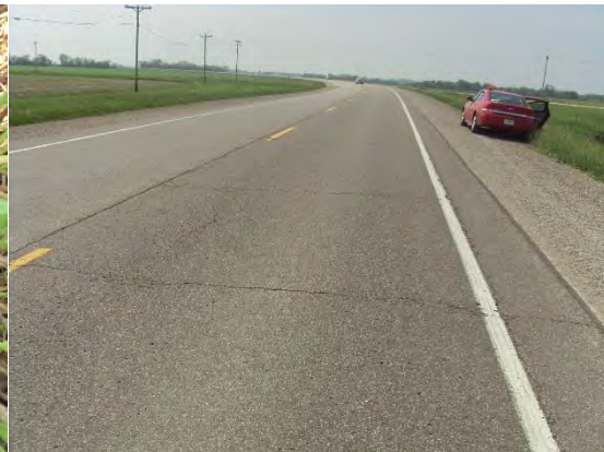
Reflection cracking
