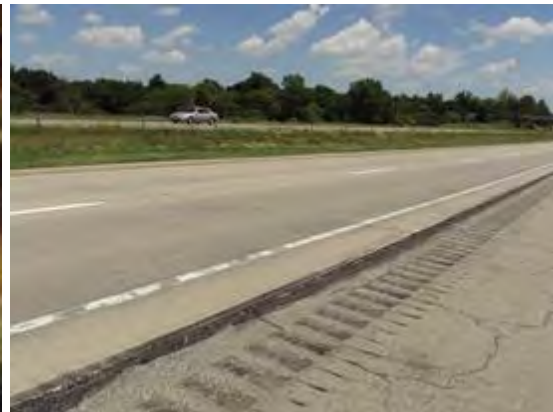
No pavement surface distress
