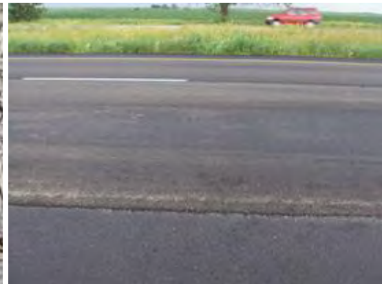
New HMA overlay
