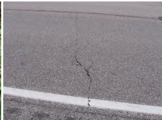
Transverse cracking
