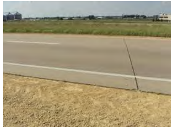
No pavement surface distress
