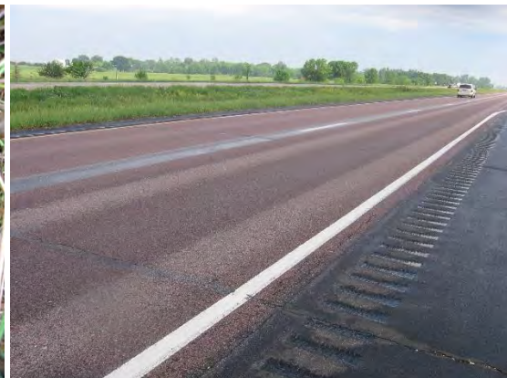
Reflection cracking
