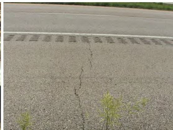
Transverse cracking
