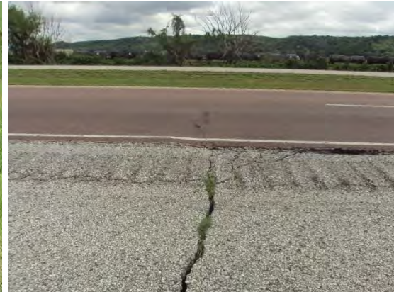
Transverse cracking/rutting
