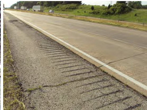
No pavement surface distress
