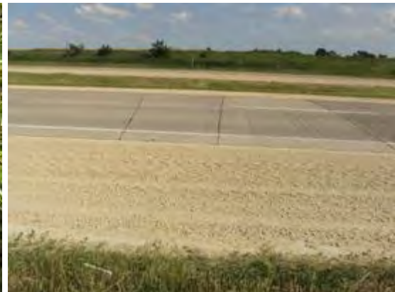
Pavement patching due to culvert
