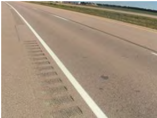
No pavement surface distress
