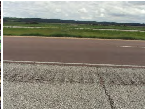
Rutting/transverse cracking
