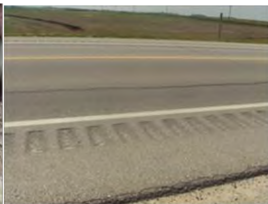
Longitudinal cracking patching
