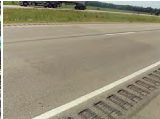
Pavement surface grinding
