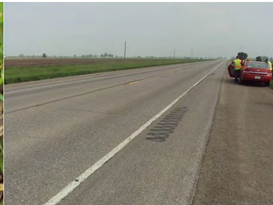
Transverse cracking
