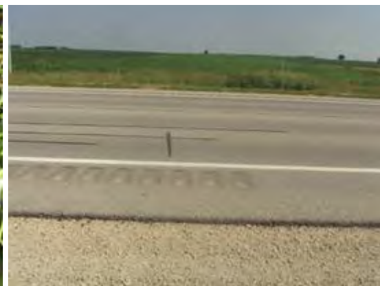
Longitudinal and transverse cracking patching
