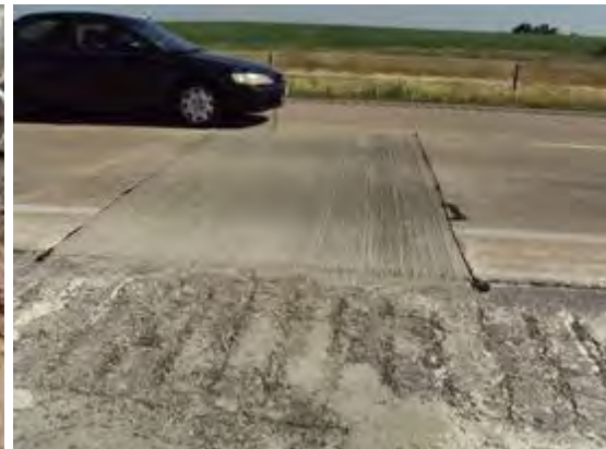
Pavement patching 50-ft. away
