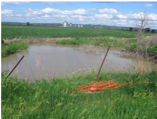
No drainage outlet
