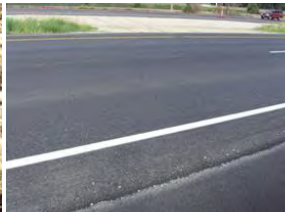
New HMA overlay
