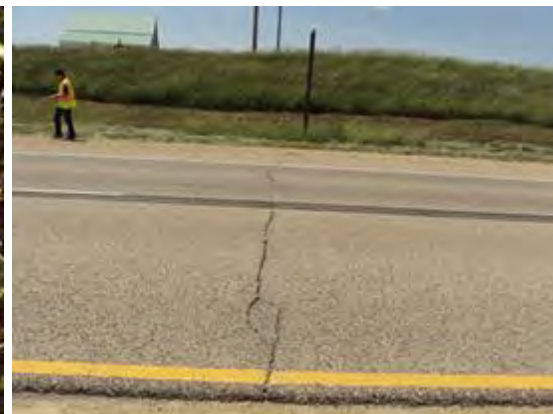
Transverse cracking
