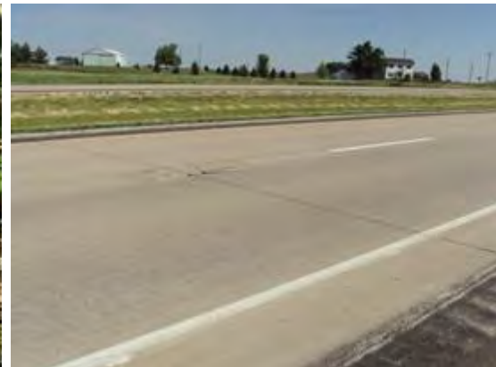
Corner crack
