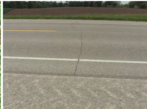
Transverse cracking
