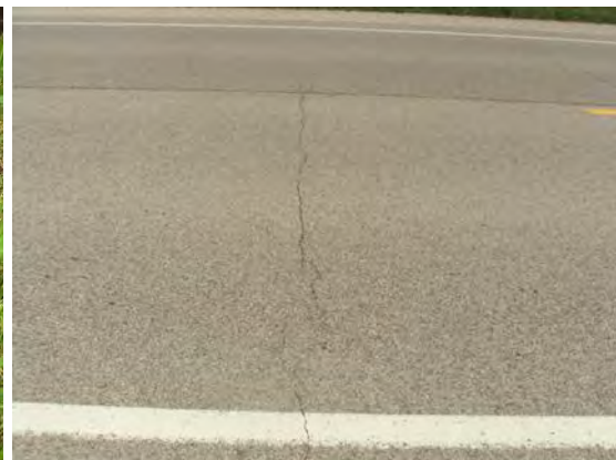
Transverse cracking
