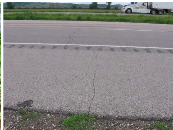
Transverse cracking
