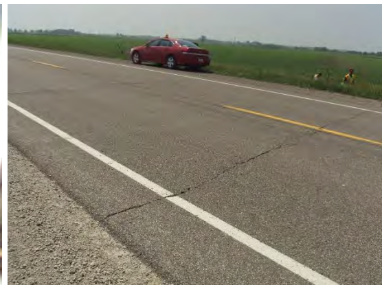
Reflection cracking
