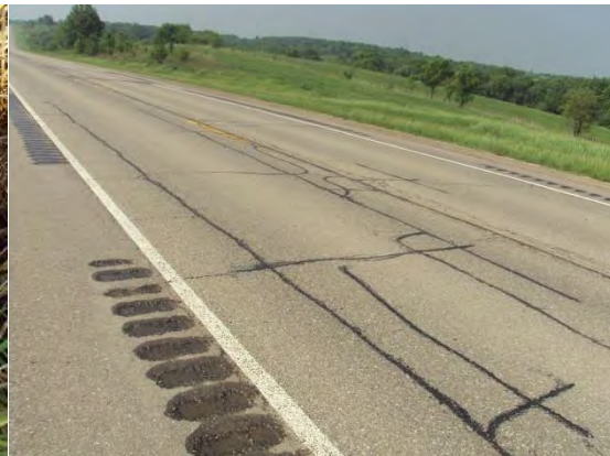
Longitudinal and transverse cracking patching
