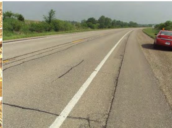
Longitudinal and transverse cracking patching
