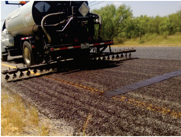
FIGURE 12 – Measuring Tack Rate and Uniformity.
