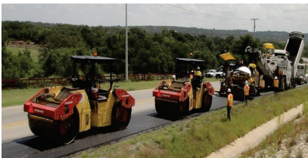
FIGURE 13 – Dual Steel Wheel Rollers Working in Tandem for Compaction.
