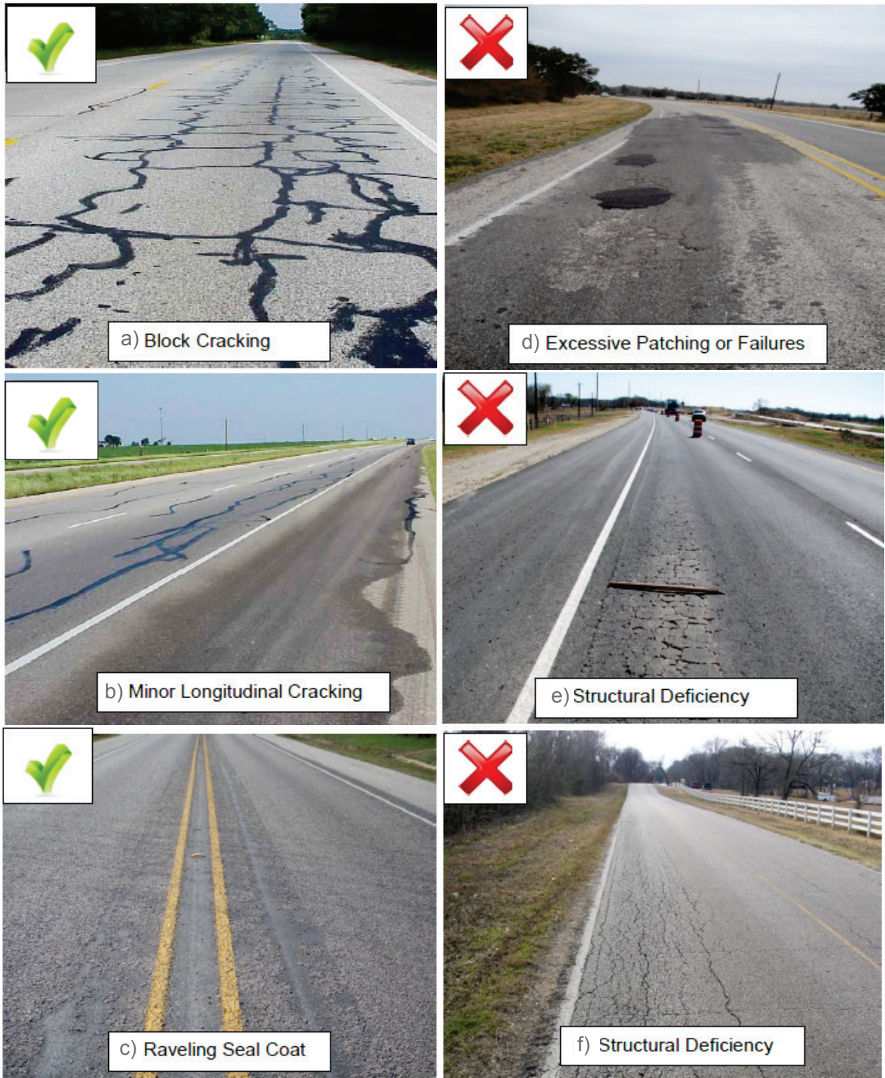
FIGURE 3 – Good and Bad Candidates for Thin Overlays.
