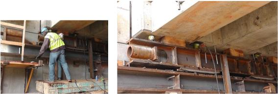
Figure 1–5 Manual jack under the fascia girder
