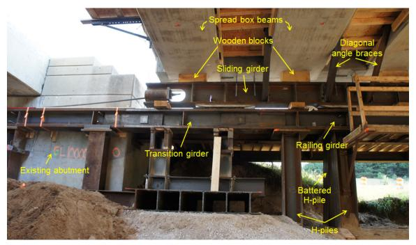
Figure 2–3 Temporary structure with new NB superstructure
