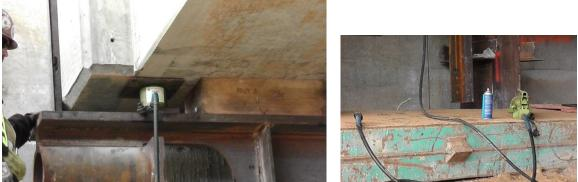
Figure 1–6 Manual jack at fascia girder and pump
