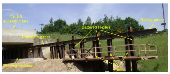
Figure 2–2 Temporary structure for NB superstructure
