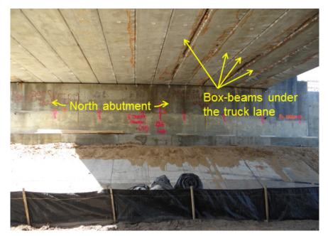
Figure 2–1 Condition of box-beams under the truck lane of old NB superstructure
