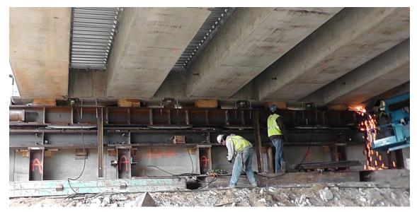
Figure 1–3 Synchronized jacks at the backwall pockets
