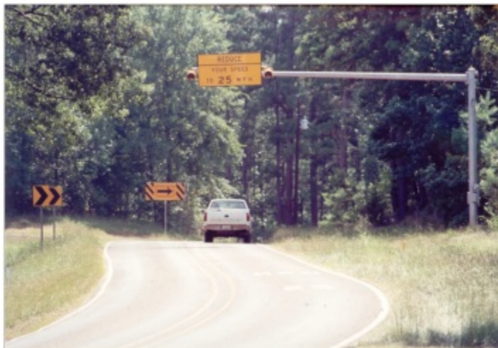
Figure 1.20: Dynamic Curve Warning System in Texas Source: Lord et al., 2011
