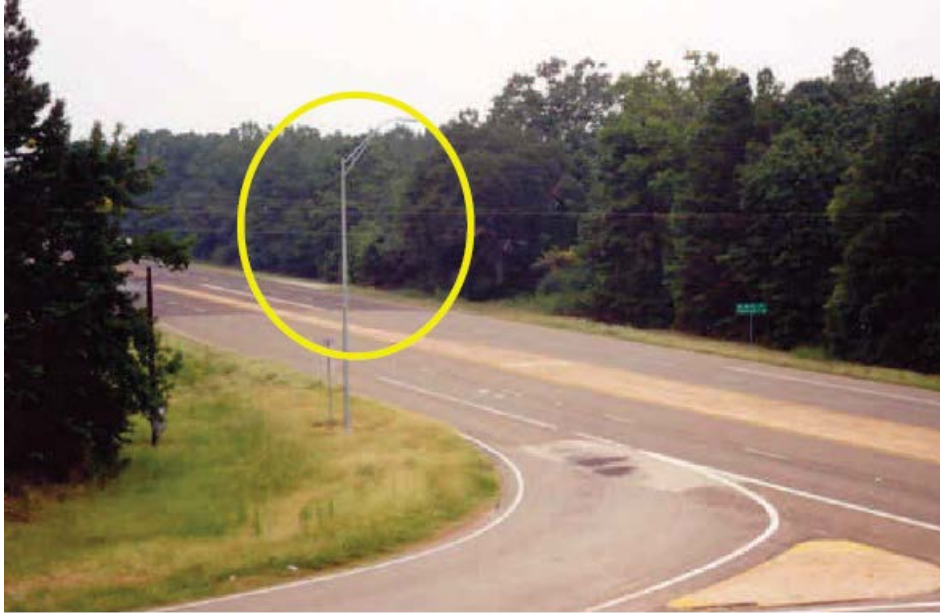
Figure 1.25: Using Lighting to Improve Visibility on a Curve
