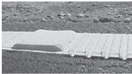
Raised Profile Thermoplastic Markers
