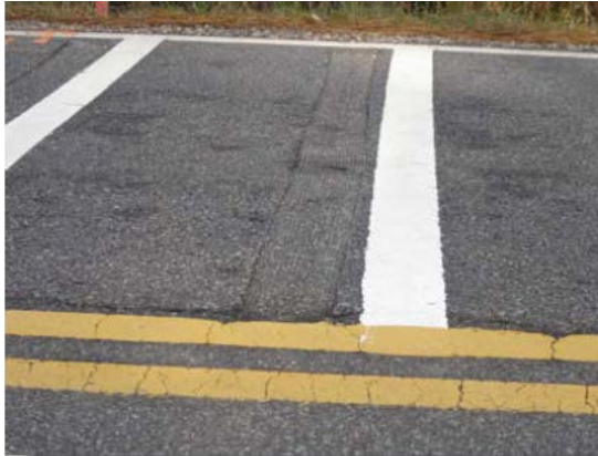
Figure 1.16: Example of Roadway Rumble Strip
