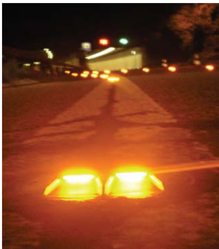
Figure 1.19: Example of Using In-Pavement LED Markers Source: TAPCO, n.d.
