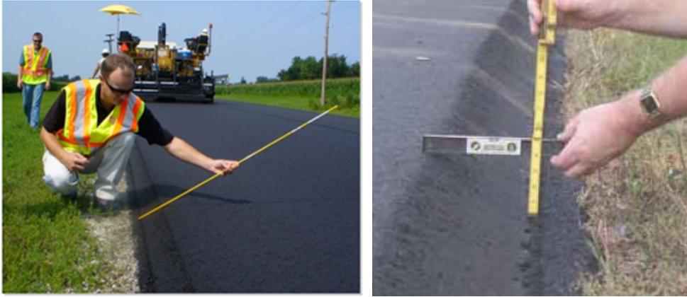
Figure 1.24: Examples of Safety Edges
