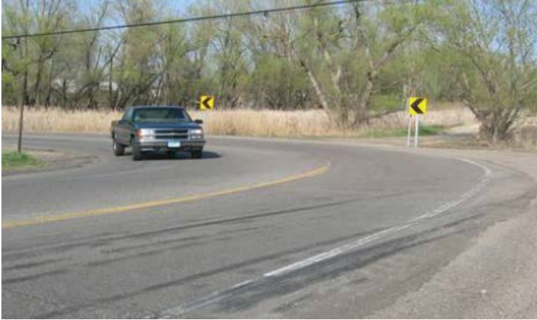
Figure 1.23: Example of Inside Shoulder Widening
