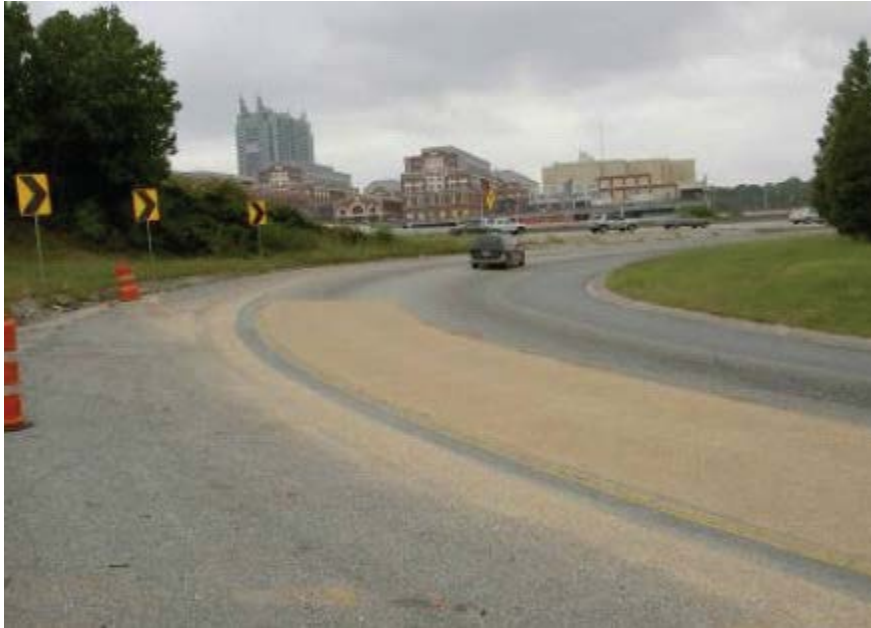
Figure 1.26: Application of Skid Resistant Material on a Curve
